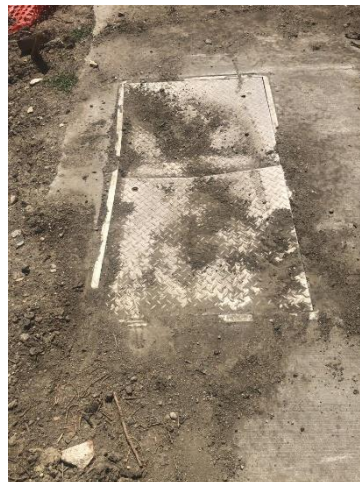
Damage to metal access cover on tunnel
