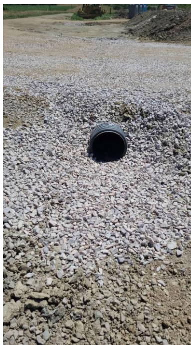
Culvert drain under the Northern entrance
