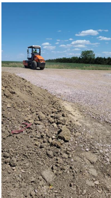
Road roller used to compact road rock
