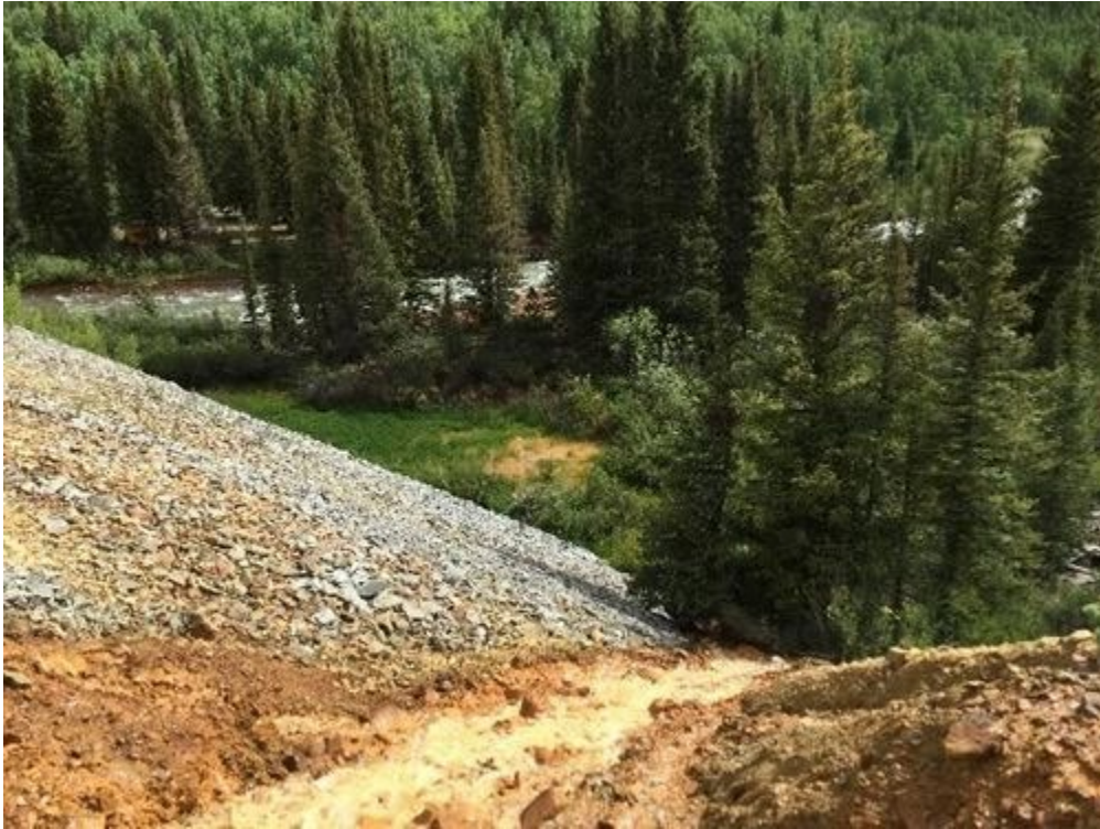
Adit flow off pile to Mineral Creek that is redirected out of constructed channel due to Beaver dam in portal
