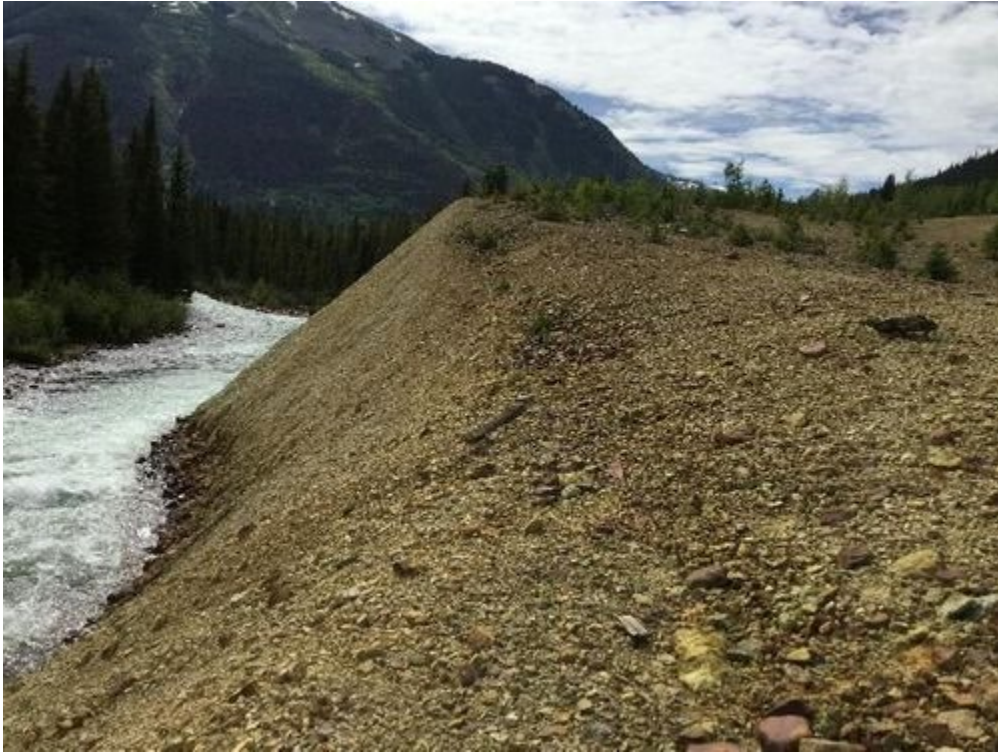
Steep Exposed Bank of Lower Pile into Mineral Crk
