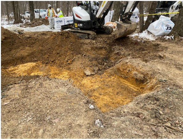
Photo No. 9; Taken on 01/28/2022 at 09:20 by START [REDACTED]. Facing N. Excavation of waste burial pit in progress, loading soil bags.
