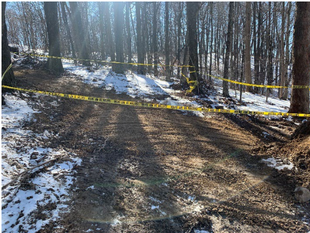
Photo No. 19; Taken on 01/31/22 at 14:21 by START [REDACTED]. Facing W. Backfilled excavation pit, with polyethylene liner, filled with pea gravel to grade surface.
