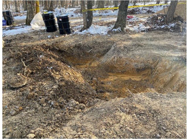
Photo No. 6; Taken on 01/27/2022 at 09:56 by START [REDACTED]. Facing Southwest (SW). Excavation of waste burial pit in progress.
