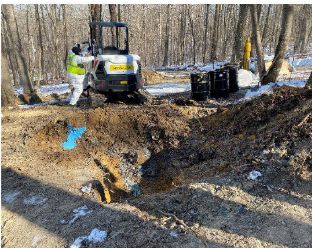
Photo No. 3: Taken on 01/26/2022 at 11:23 by START_ [REDACTED]. Facing East (E). Paint waste visible within the soils of the pit.
