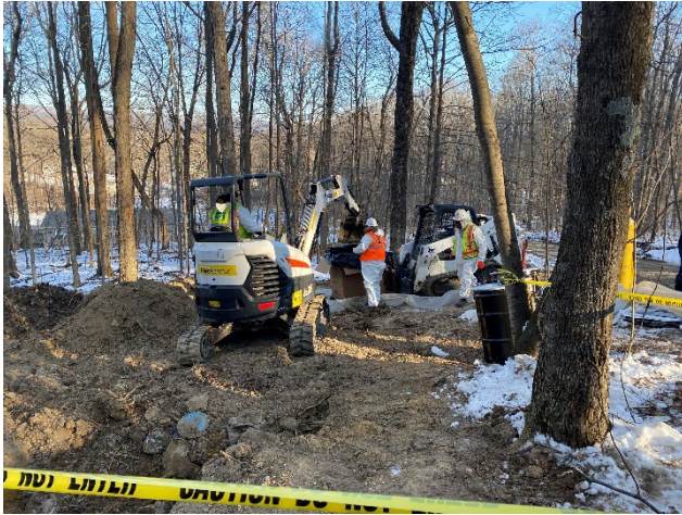
Photo No. 5; Taken on 01/27/2022 at 09:13 by START [REDACTED]. Facing North (N). Filling cubic yard bags with soils.
