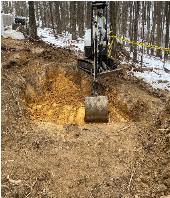
Photo No. 11; Taken on 01/28/2022 at 13:16 by START [REDACTED]. Facing SW. Excavation of waste burial pit in progress, loading soil bags. Less impacted soils can be seen.
