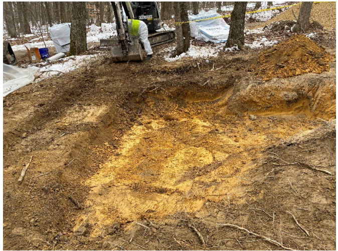
Photo No. 10; Taken on 01/28/2022 at 11:07 by START [REDACTED]. Facing E. Excavation of waste burial pit in progress, loading soil bags, and removing waste paint containers from soils.
