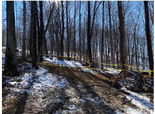
Photo No. 20; Taken on 01/31/22 at 14:21 by START [REDACTED]. Facing W. Backfilled excavation pit, with polyethylene liner, filled with pea gravel to grade surface.
