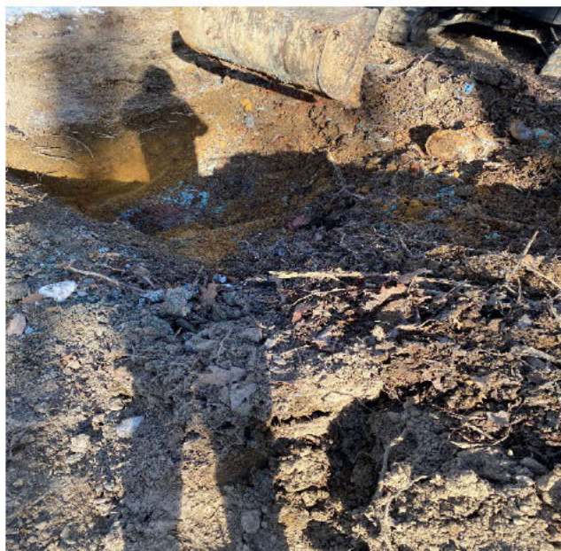
Photo No. 2: Taken on 01/26/2022 at 10:44 by START_ [REDACTED]. Looking down at pit. Blue and red paint waste visible within the soils of the pit.
