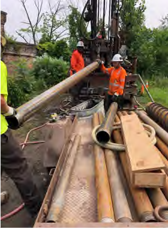
Installation of Permanent Casing at Well HF-130
