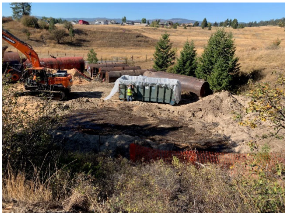
Adding poly liner to roll-off box #4
