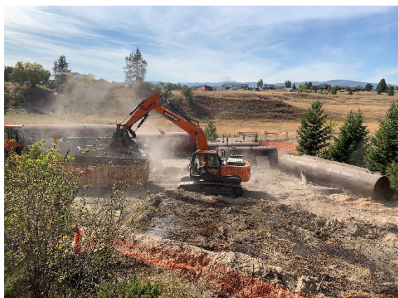
Loading scrap metal from tank #6 and #7
