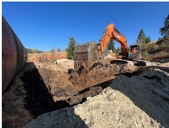
Stablizing hydrocarbon waste with sawdust
