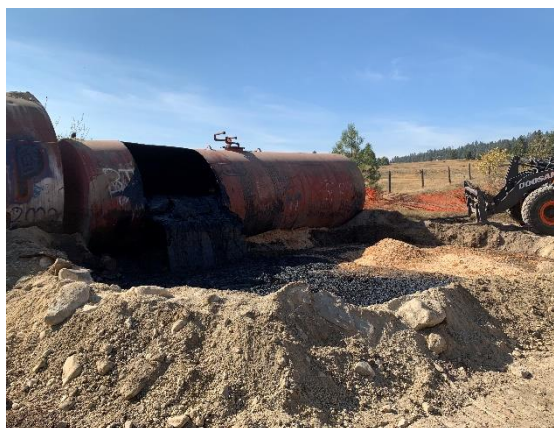
Tank #13 drains in solidification pit
