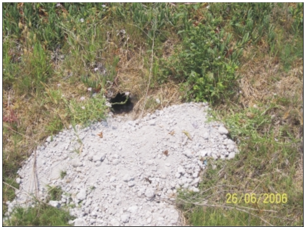
Photo 18: Waste material extracted from under the soil cover by burrowing animals. Photo by A. Rice.
