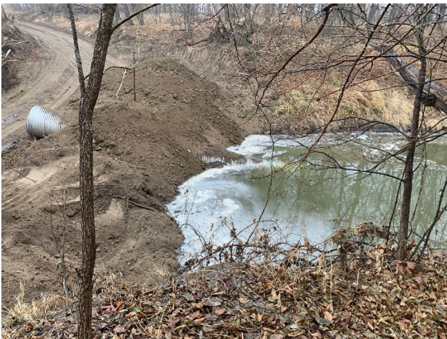
An earthen underflow dam constructed to prevent further migration of oil. (Public domain photo by EPA)
