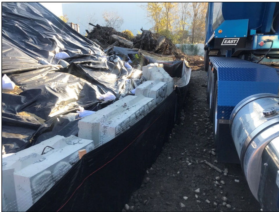
Photo #6: Looking east along southern end of Pile B with silt fence installed.
