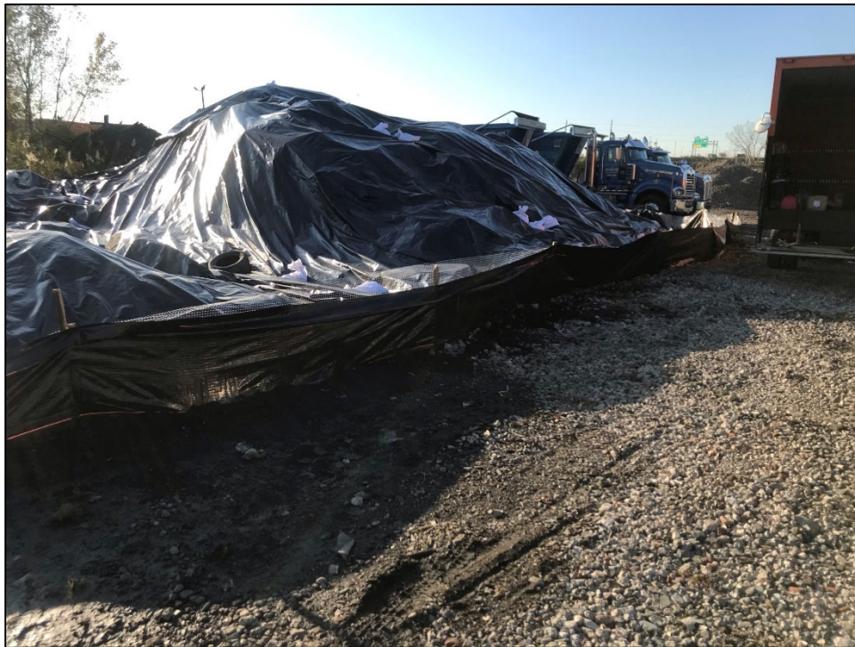
Photo #5: Looking SE at western side of Pile B with silt fence installed.
