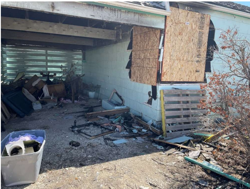
Asbestos containing siding is falling off property onto the ground.
