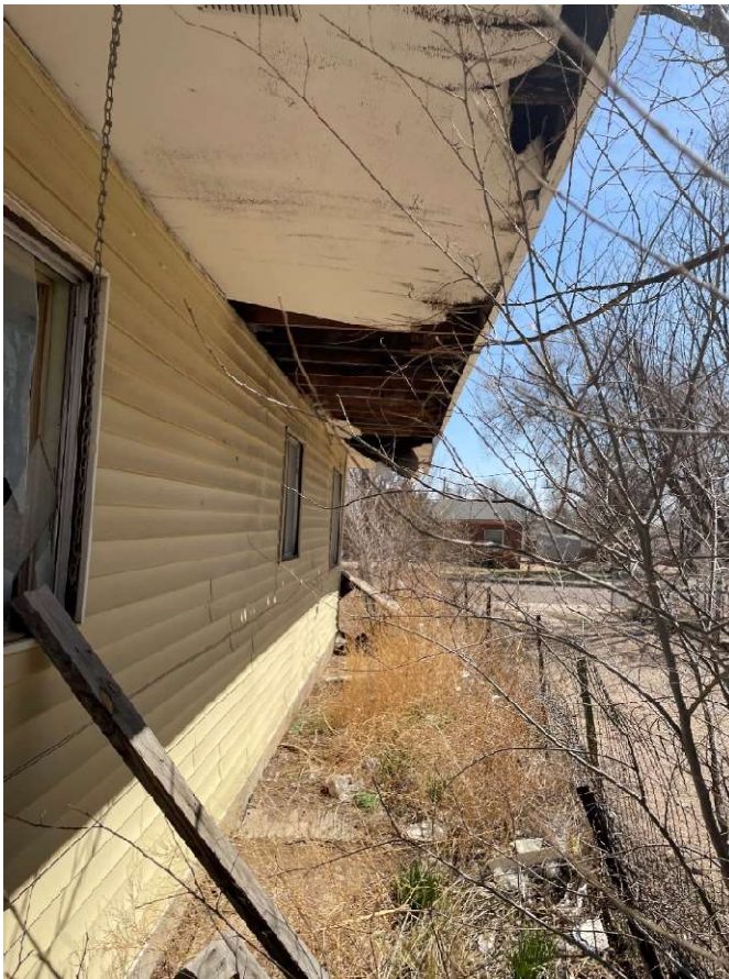
Front of property. Note roof is separating creating openings into house. The roof contains ACM.
