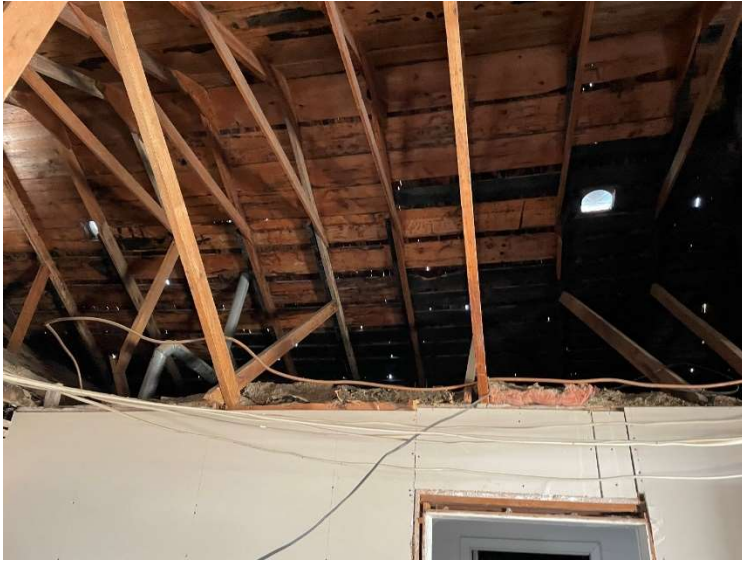
Roof supports is missing, and many holes observed in roof of property.
