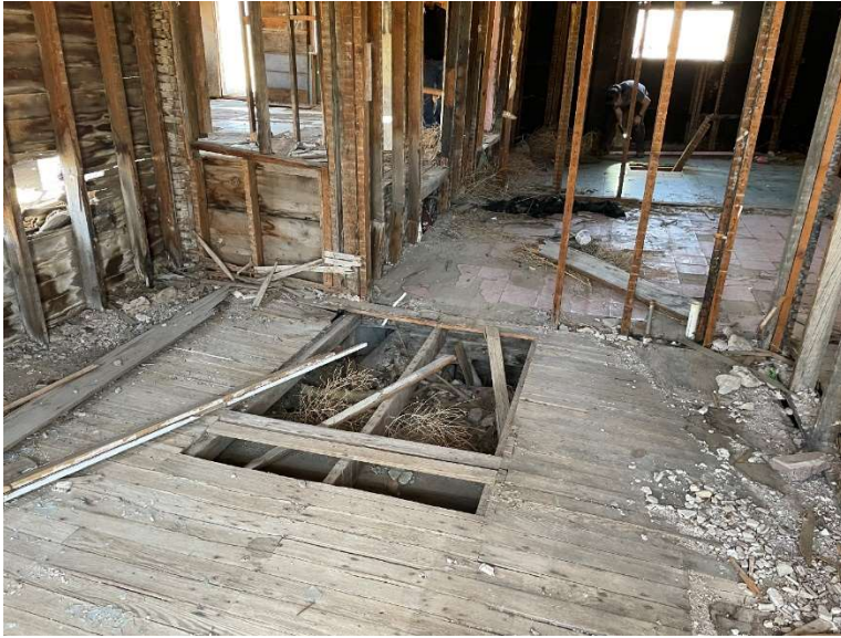
Multiple large holes in the floor and walls.
