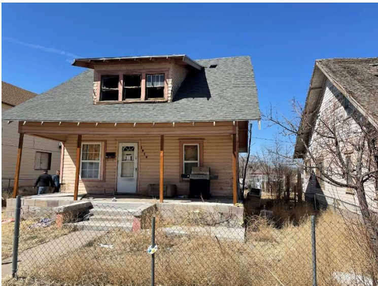
Front of 1010 Raton Ave. Holes in roof were created by fire department during last fire. Floor inside is about to collapse from all the water damage from fires.
