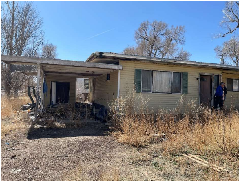
Front of property. Note roof is separating creating openings into house. The roof contains ACM.
