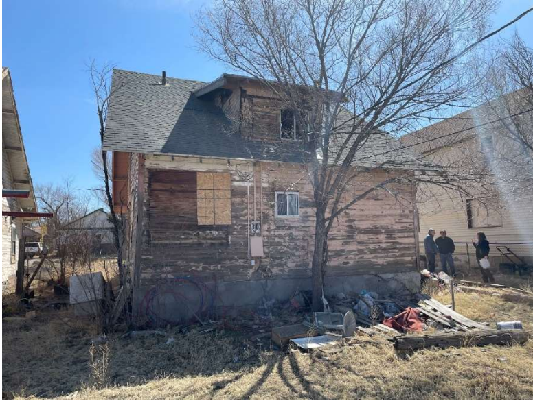
More holes in roof were noted on this side of roof from fires.
