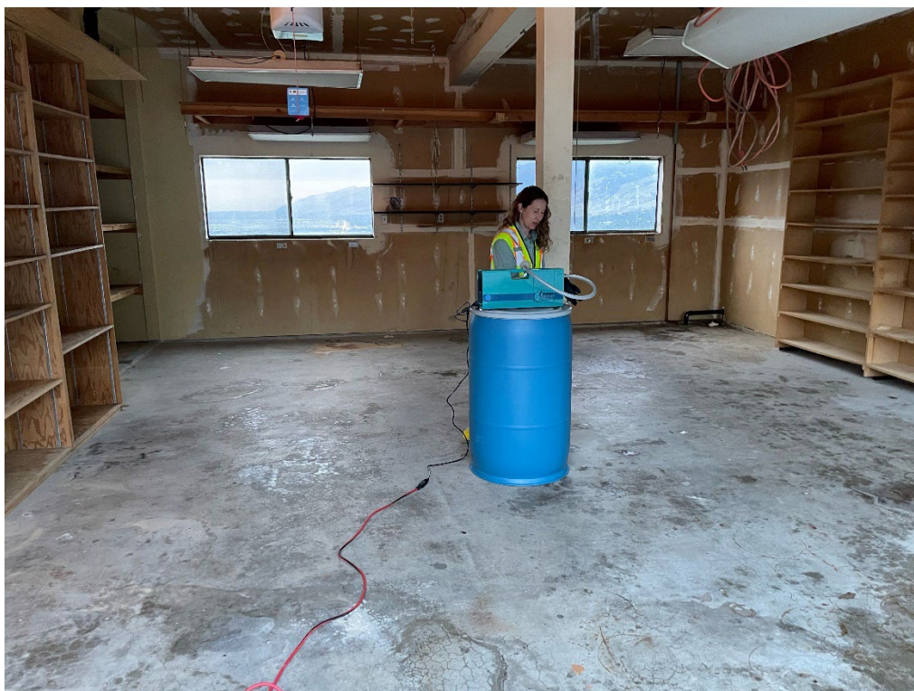
Setting up clearance air monitoring run.
