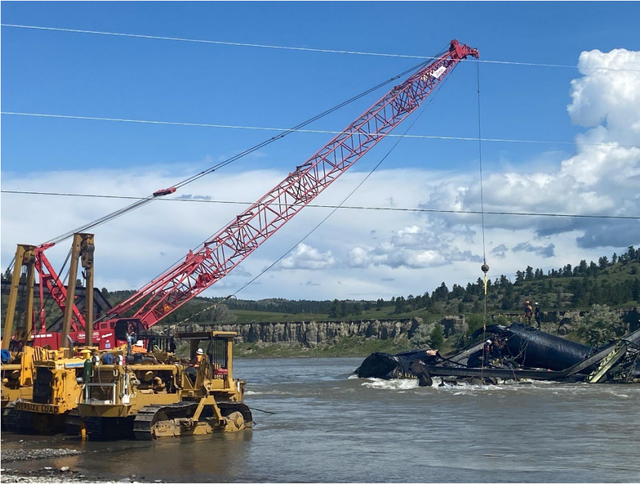
Crews rigging a railcar for removal from river.
