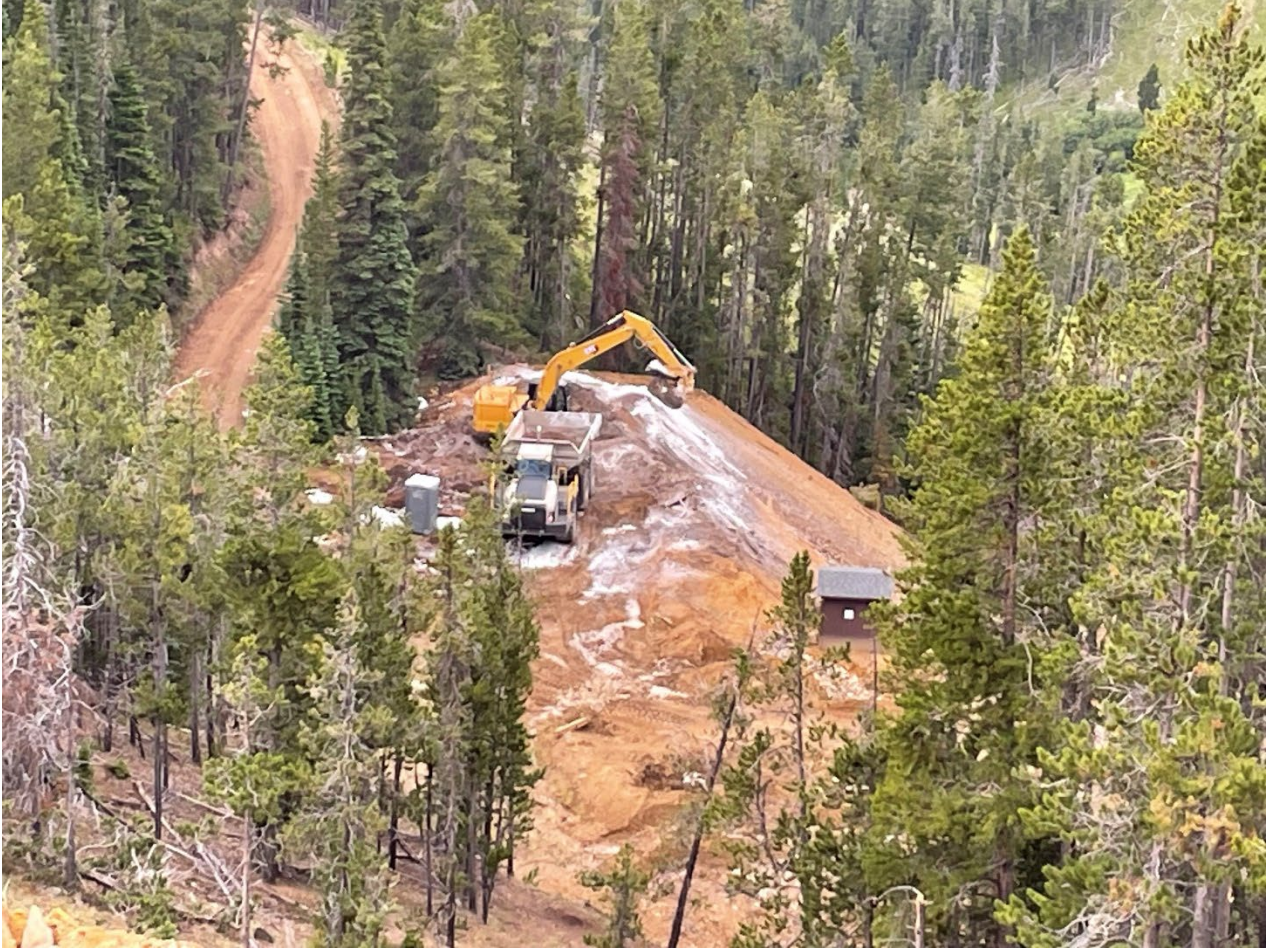
Excavator loading waste rock below the Silver Dyke adit.
