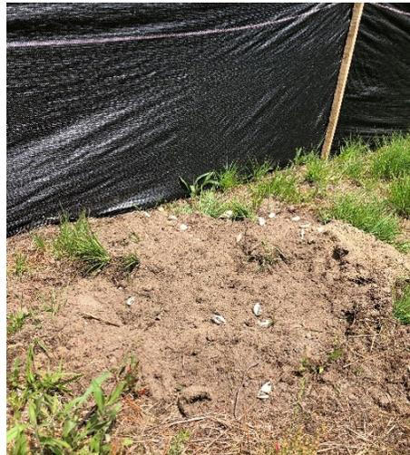
Silt Fence installed on site to keep turtles from entering the work zone. The silt fences are working, as a turtle's nest was found next to the fencing.
