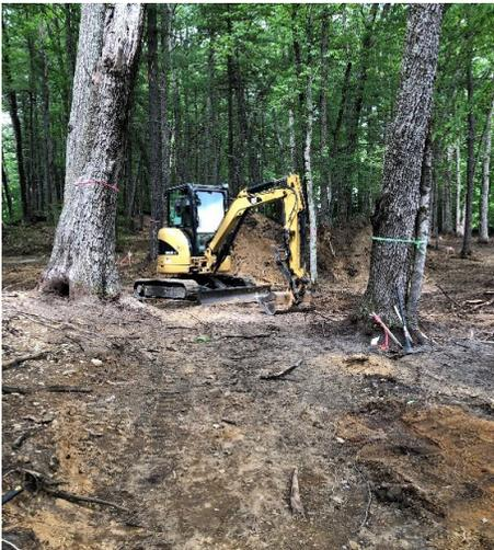
A foot of contaminated soil was excavated from the site. Once excavation is complete a nonpermeable sheet will be installed and clean topsoil will be placed on top.
