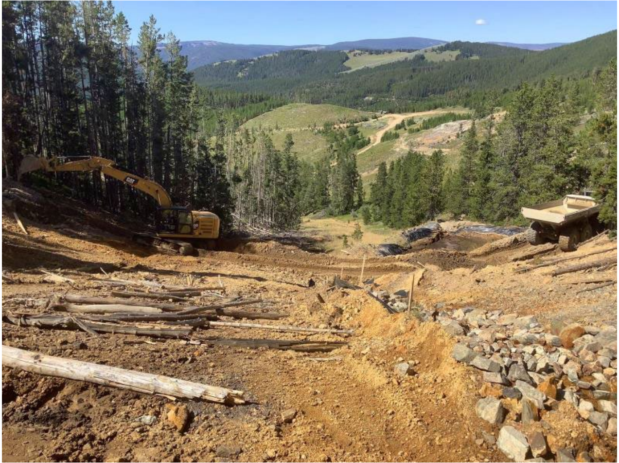
Slope stabilization below adit where EPA is working. Logs are being added for slope stability.
