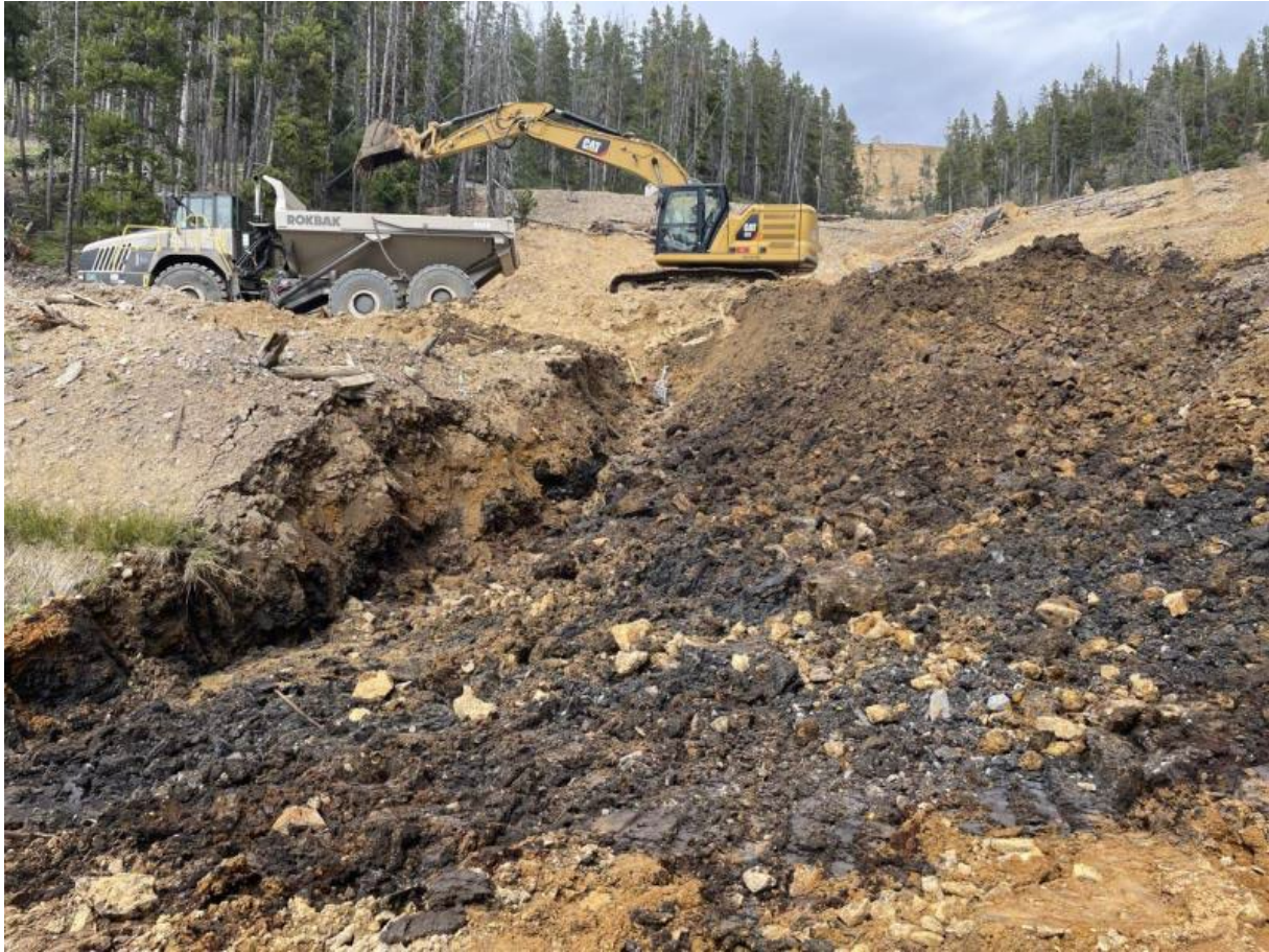
Excavating mine waste to create a water management pond, looking up towards the adit.
