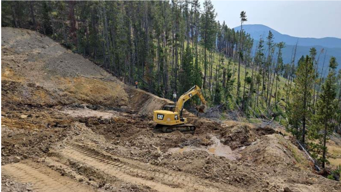
Containment pond berm construction.
