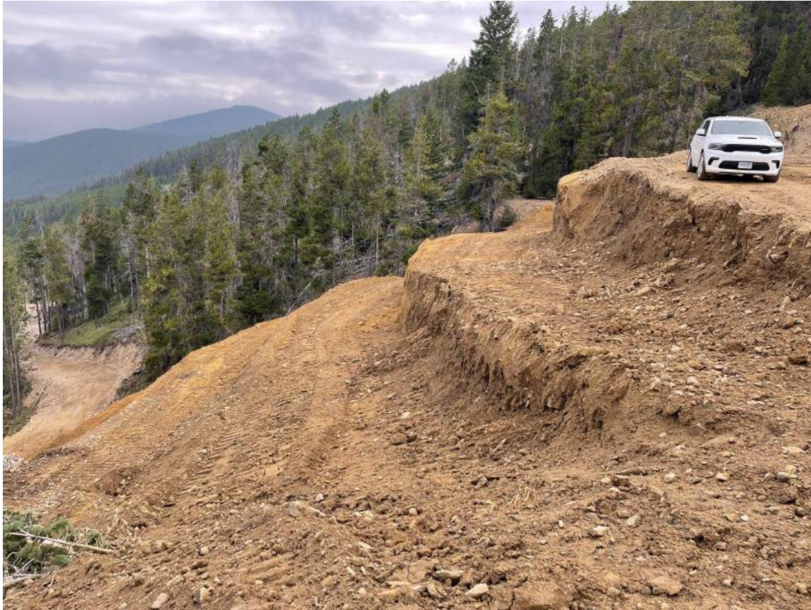
Erosion benches above the adit.
