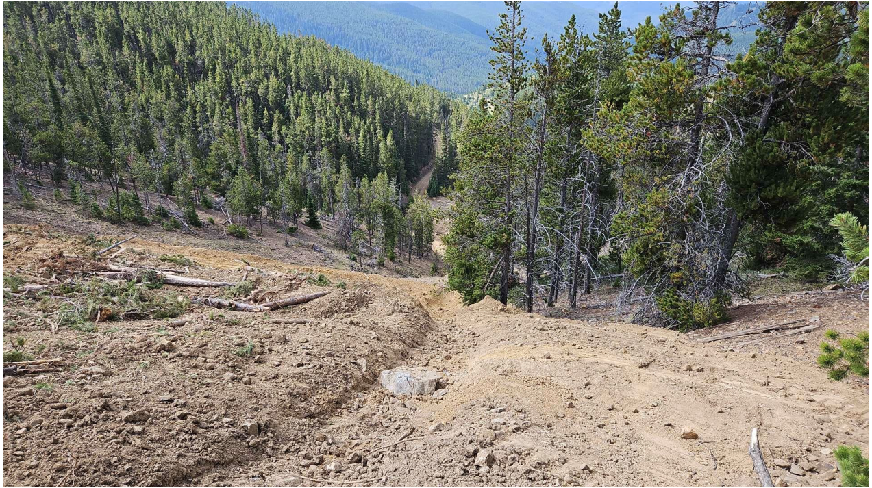
Channel along West side of benches above adit to divert surface water runoff away from adit. Channel will eventually be lined with rip-rap.
