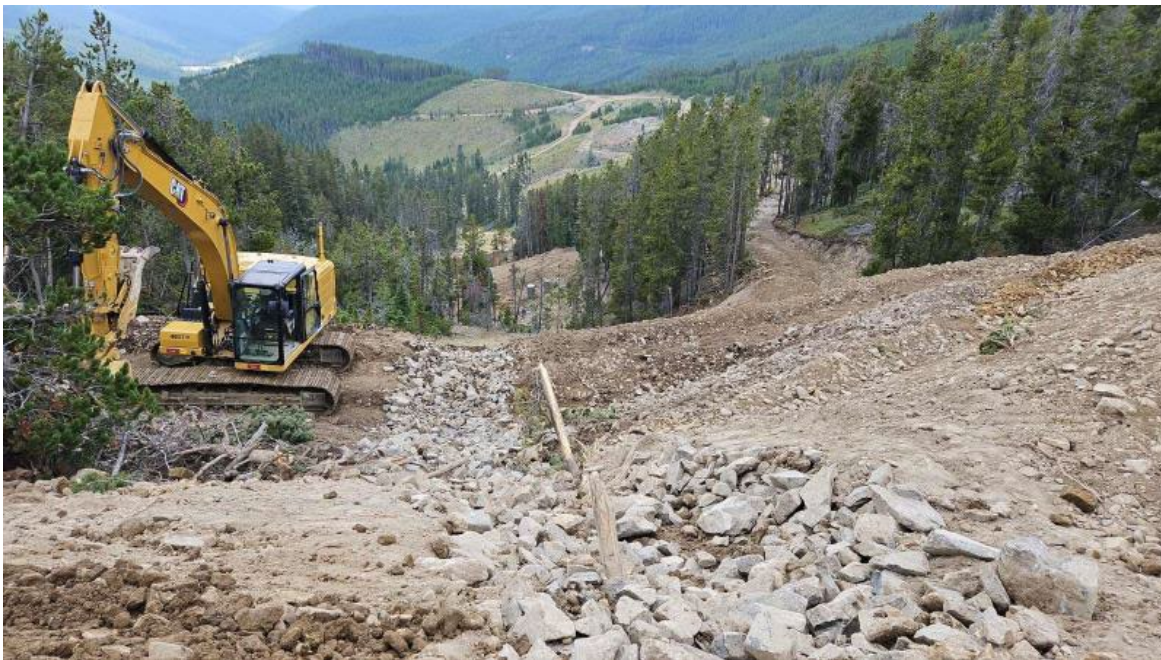
Rock-lined channel on East side of benches.
