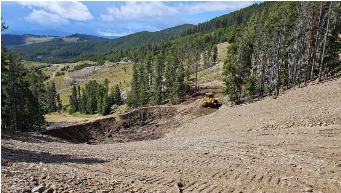
Lower retention pond, capacity increased to hold over 160,000 gallons.
