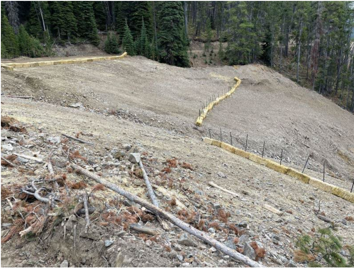
Drainage controls (hay bales) placed on restored slope below adit to aid erosion control.
