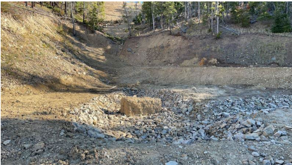
Upper retention pond, outside adit, has been removed and the area has been regraded and partially lined with rock.
