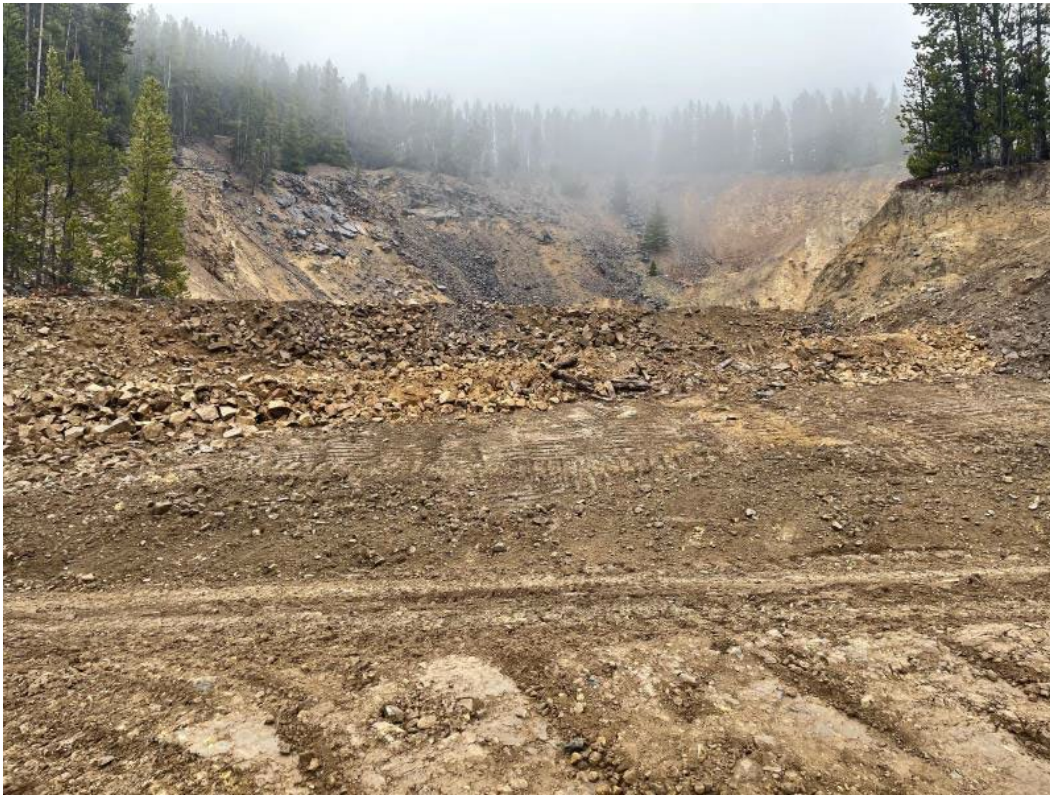
Berm and ditch installed to protect public safety and prevent vehicular access to the Glory Holes.
