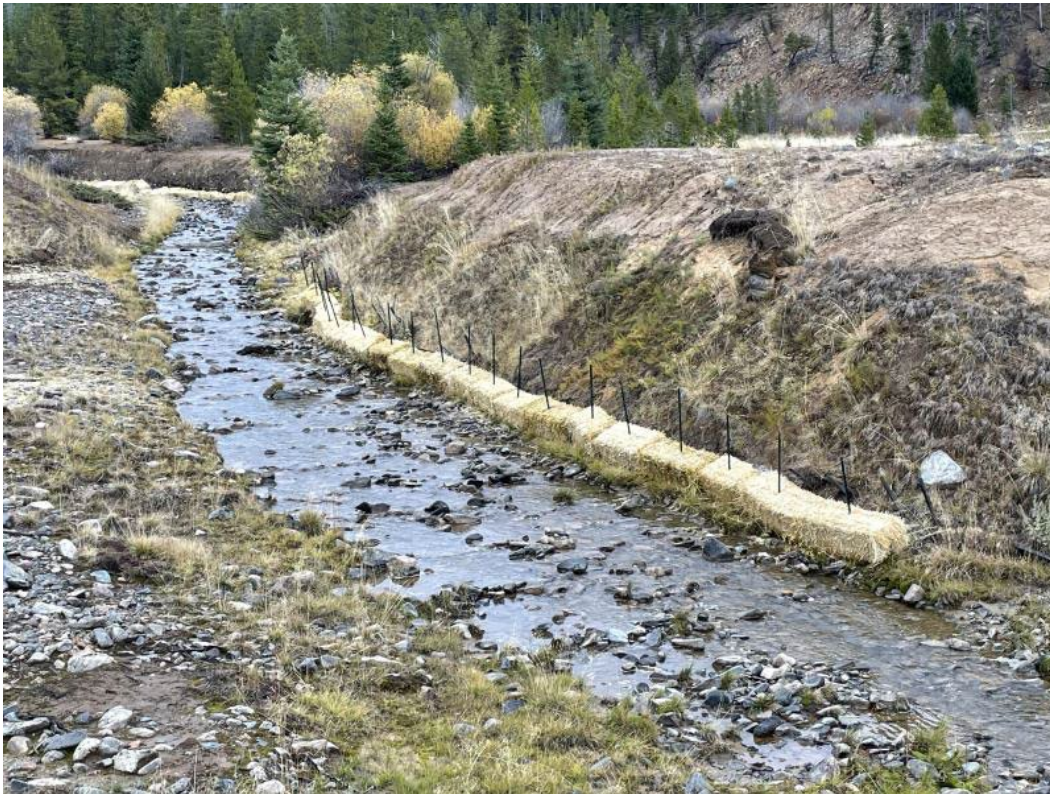
Replacement of hay bales along the toe of the tailings in Carpenter Creek.
