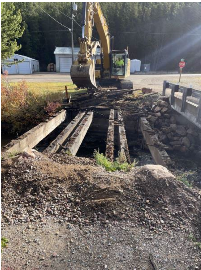
O'Brein street bridge over Belt Creek removal.
