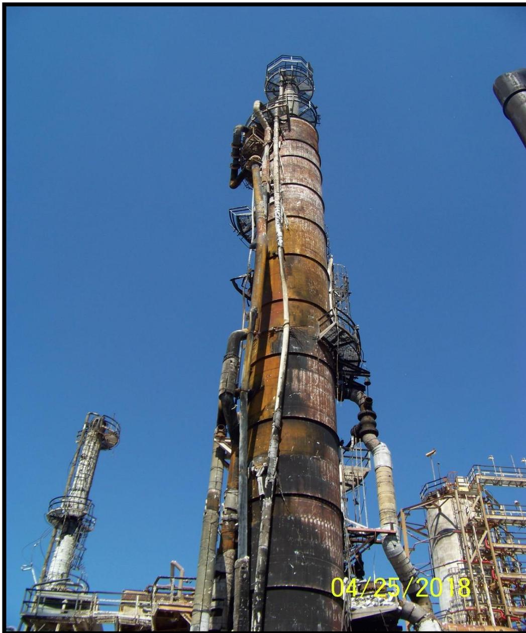
**Expanded view of the Fractionator Tower and fire damage to associated feed / return piping**
