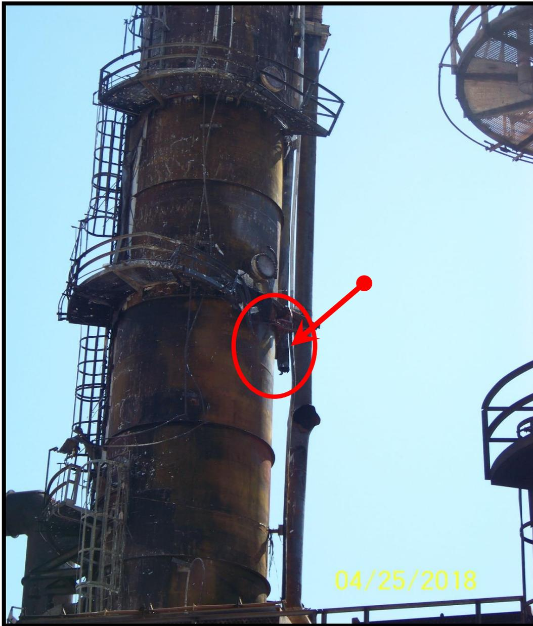
**Photo of the Main Fractionator tower and point of rupture of the 10" feed piping**
