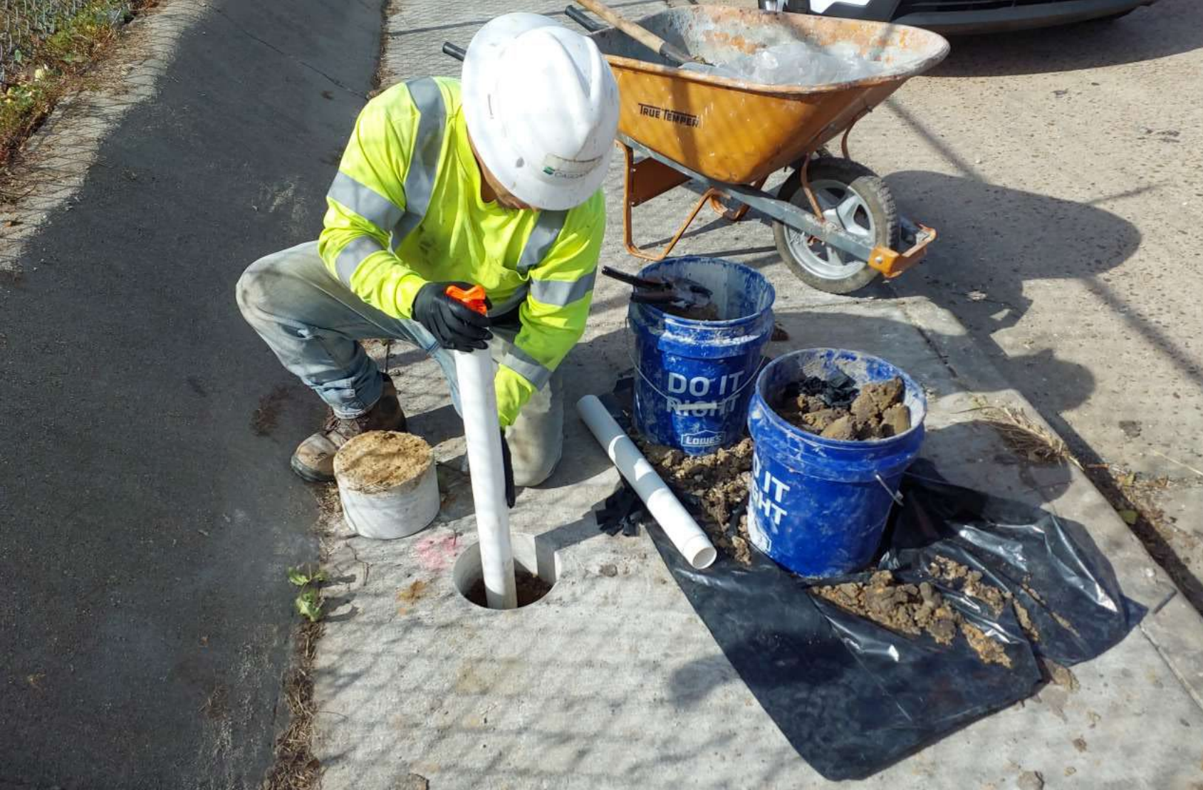
Groundwater Monitoring Well Installation Liberty Rd
