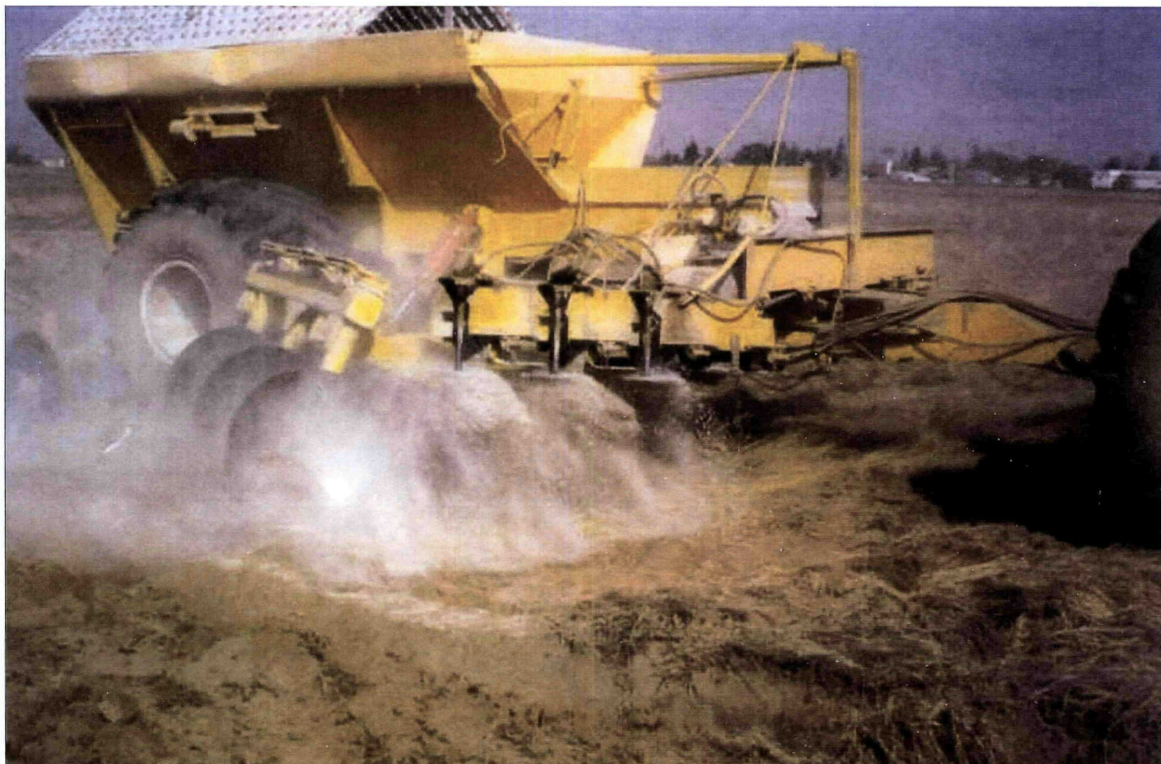
Photograph 2-9. Close-up of Tilling with Lime Amendment
