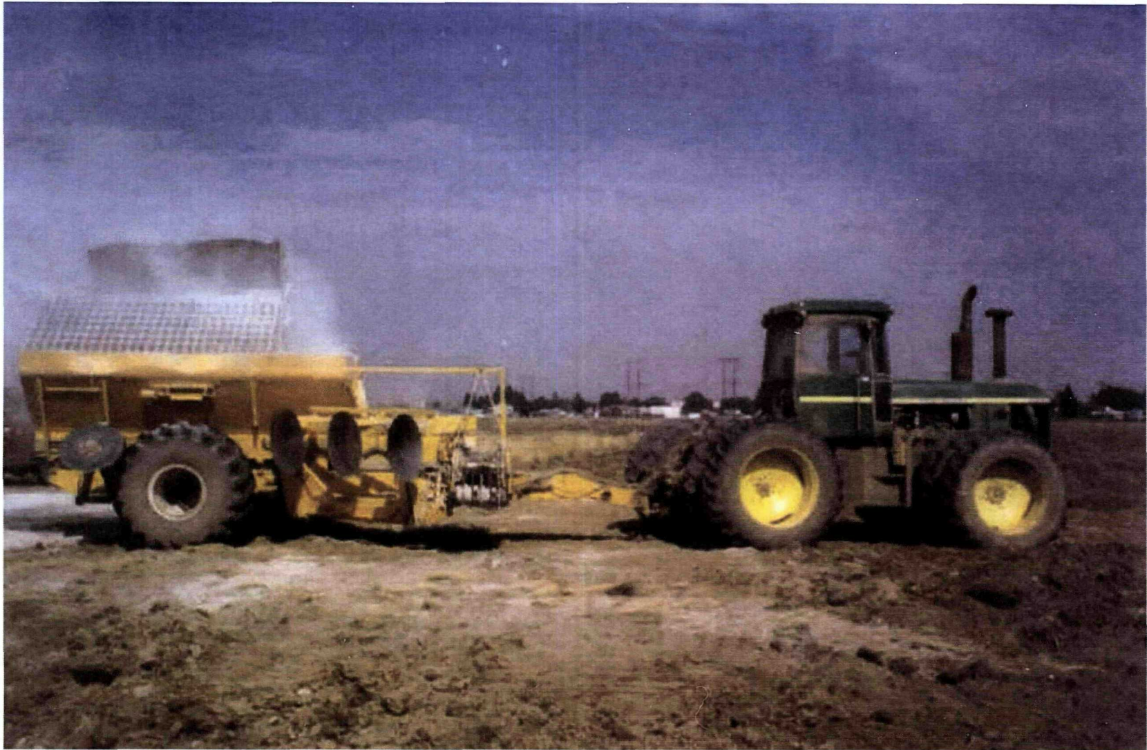
Photograph 2-8. Tilling with Lime Amendment
