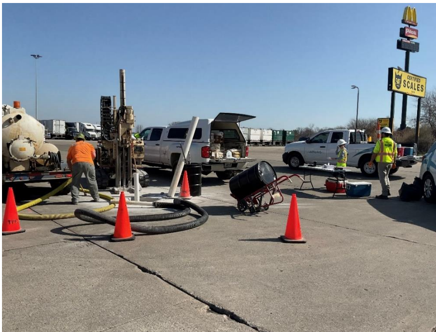
On-site subsurface investigation to determine the extent of contamination. Investigation includes soil sampling, groundwater sampling, and installing product recovery wells on April 9, 2024.
