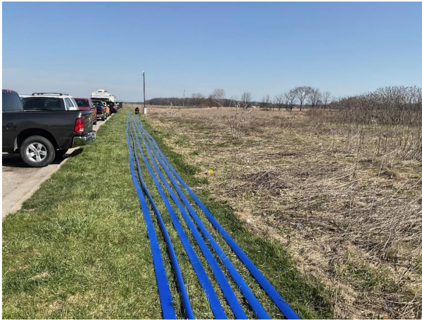
Hose line prepared to discharge treated wastewater from the on-site water treatment system, known as the granulated activated carbon system on April 9, 2024.
