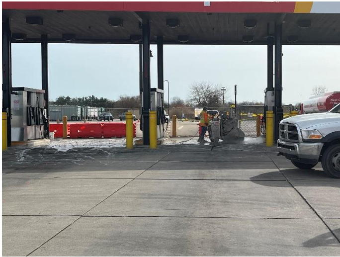
Duffey conducting concrete cutting activities at diesel pumps island
