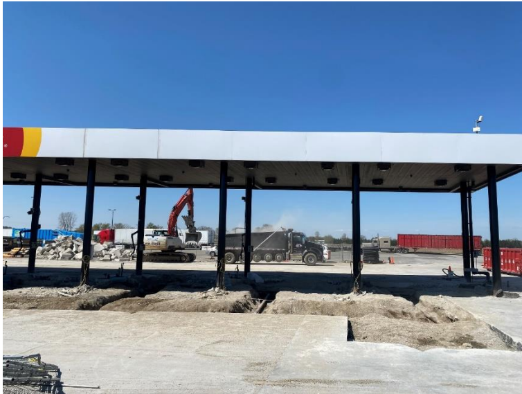
Dismantling the on-site diesel fuel system and removal of contaminated gravel/soils, April 22, 2024
