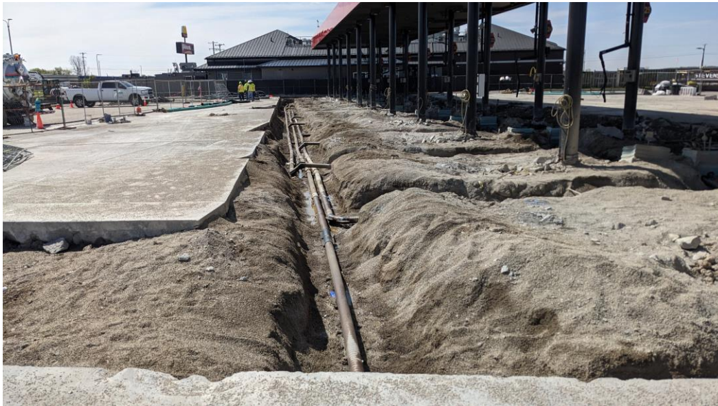
Uncovered on-site diesel fuel system and product line trenches, April 25, 2024
