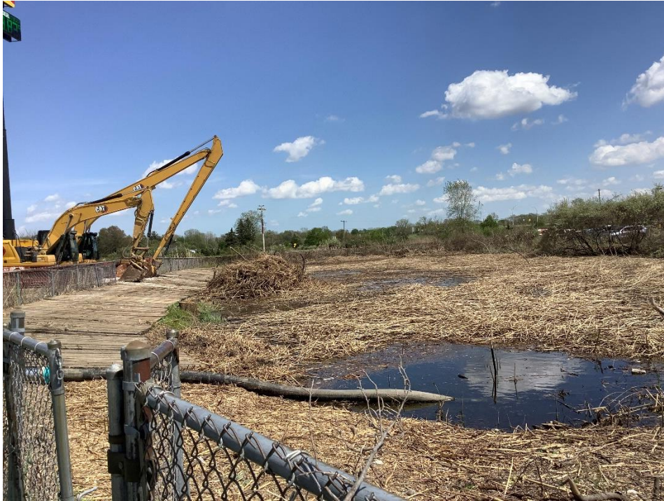
De-watering the on-site retention pond.
