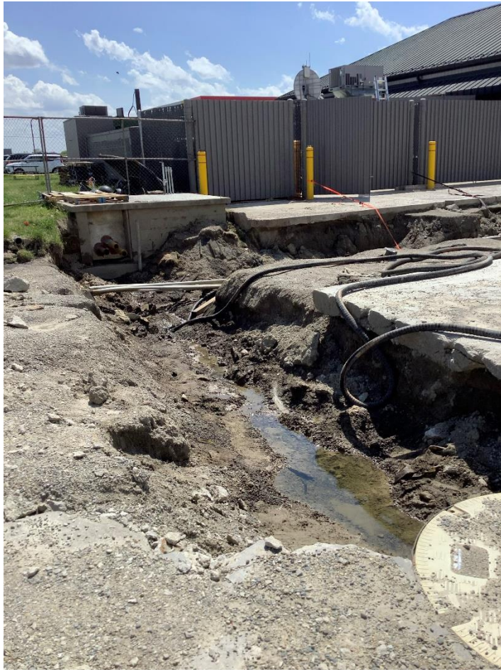
Active recovery of oil/water mixture from drain backflow in the excavation near the pumps.
