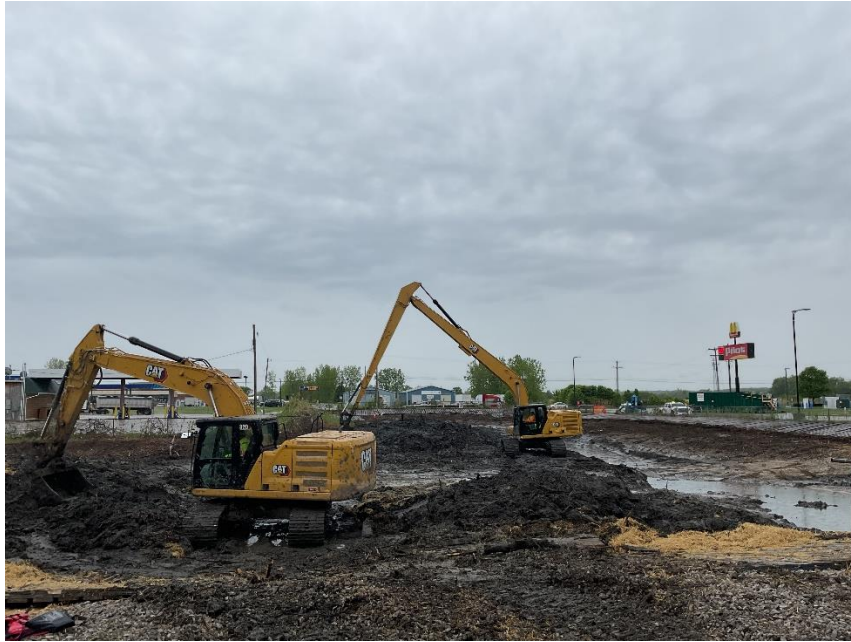
Excavation of the on-site retention pond.
