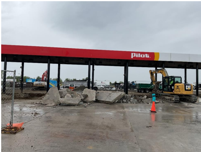
Excavation of concrete, gravel, and soil in the rear parking lot.
