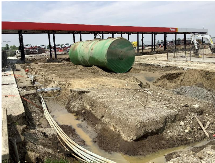
Biodiesel tank removed from excavation
