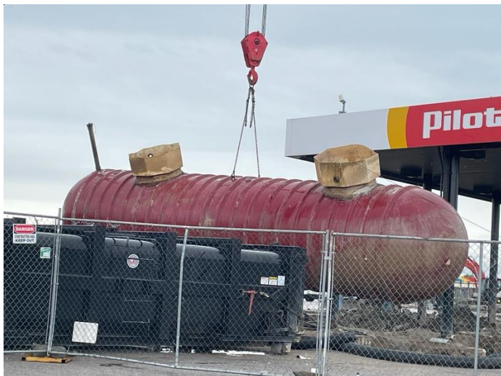
DEF tank removed from excavation
