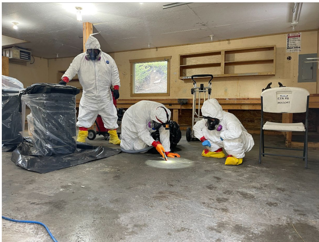
Working hard to vacuum beads of mercury in cracks.
