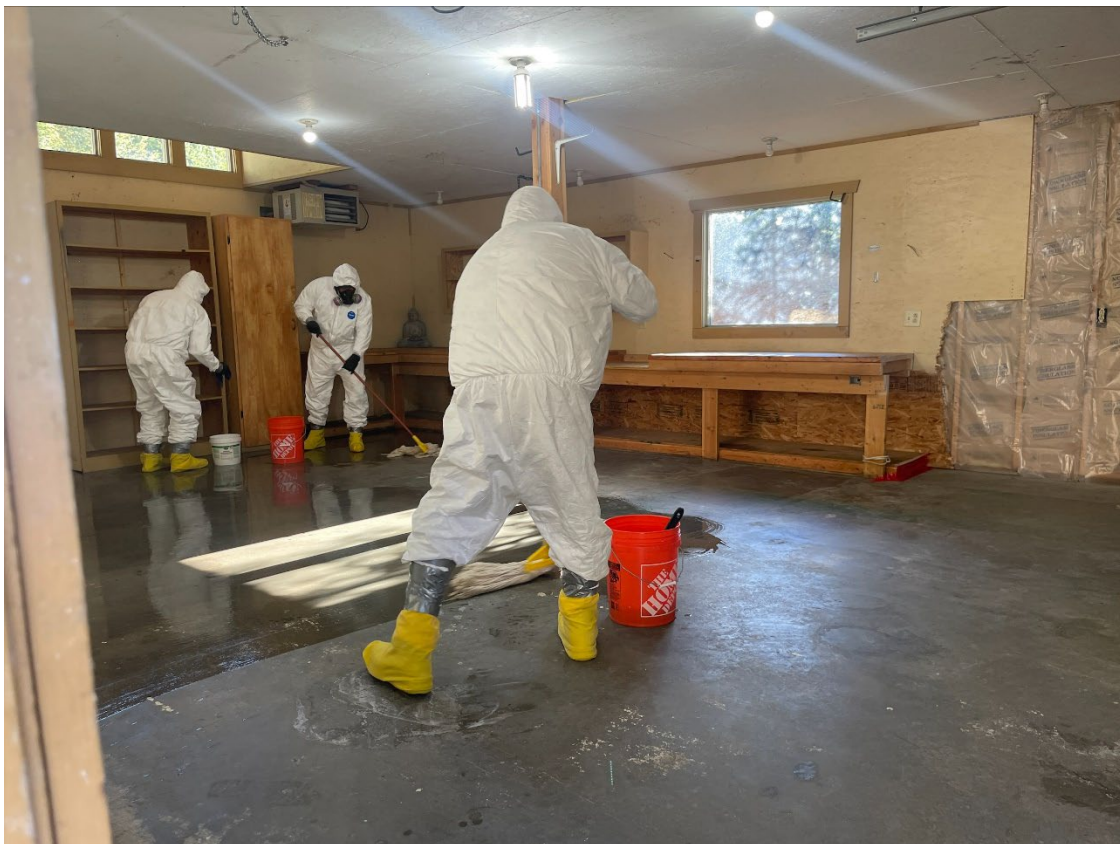
Application of HgX to interior of garage.
