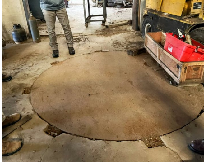
Figure 4: View of the cap to an underground storage tank in Building 2 with cracks in the cement.
