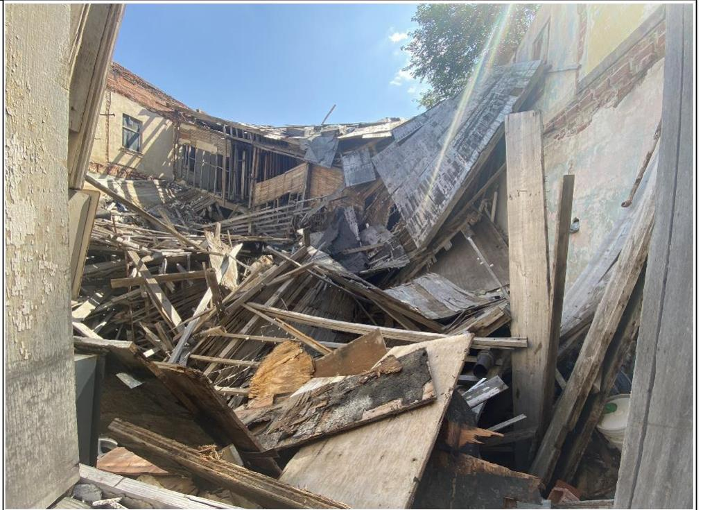
CDPHE consultant Vertex photos 8-7-2023. Top photo shows second floor has completely collapsed.
