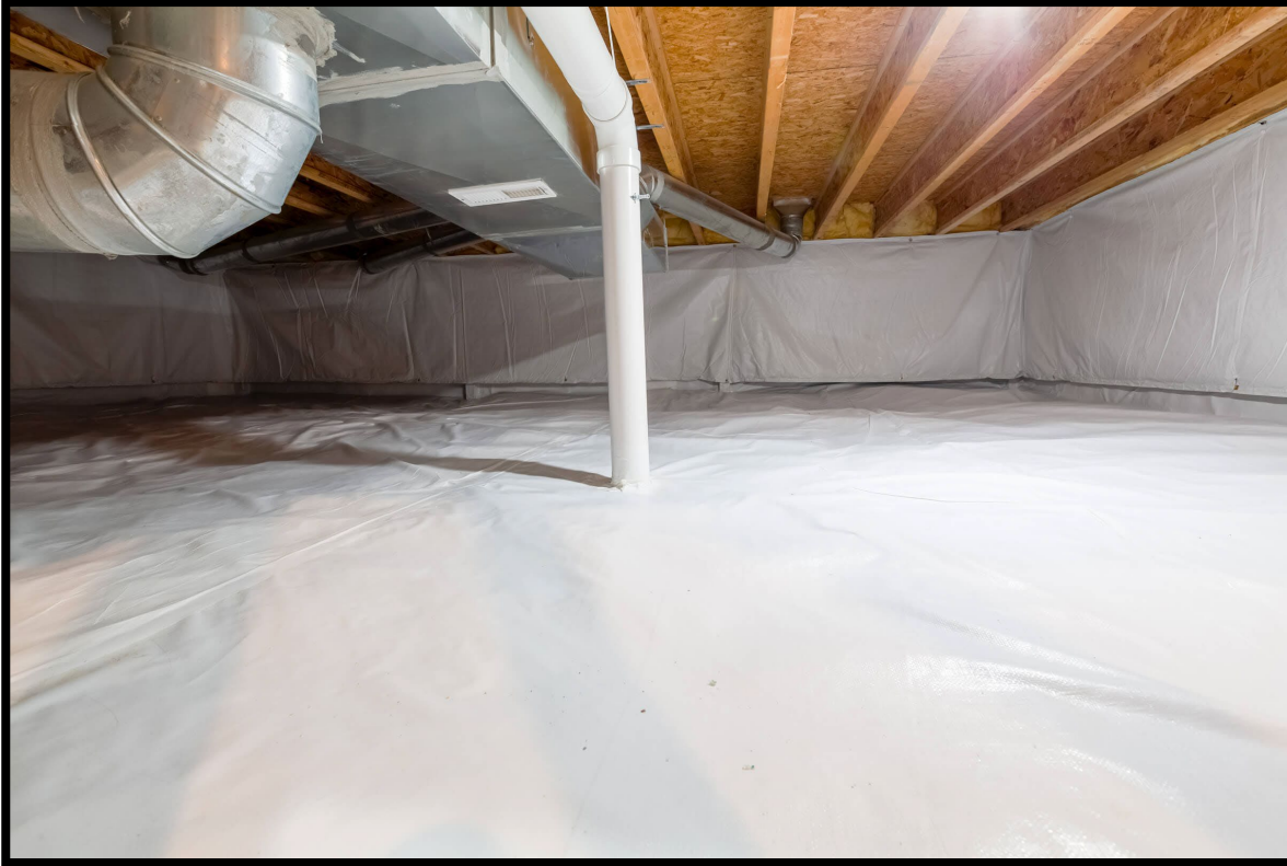
Figure 1. Example of a vapor barrier with exhaust pipe. Source: radonsolutions.com/crawlscaping
