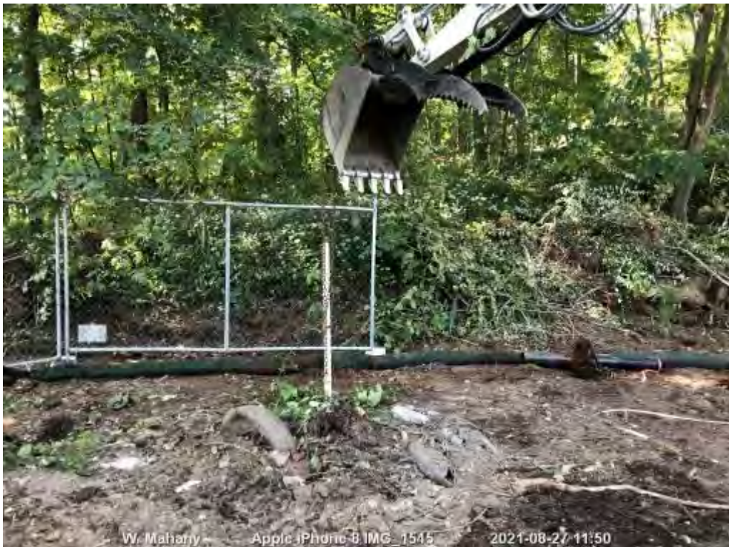
SCENE: View of groundwater monitoring well decommissioning in the southeast portion of the Site. Photograph taken facing south.
