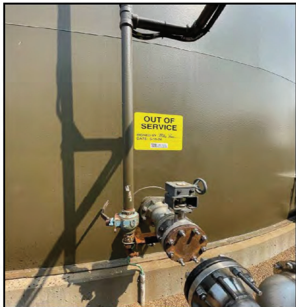
#7 - Disconnected/Isolated Lines & "Out Of Service" South View
