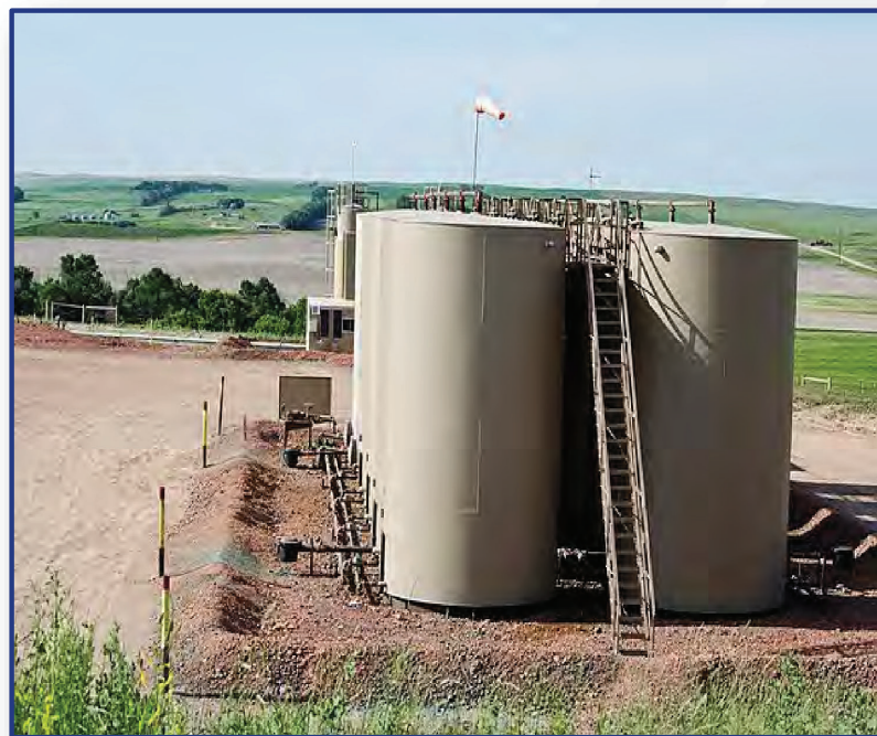
Sized Secondary Containment for Bulk Containers
