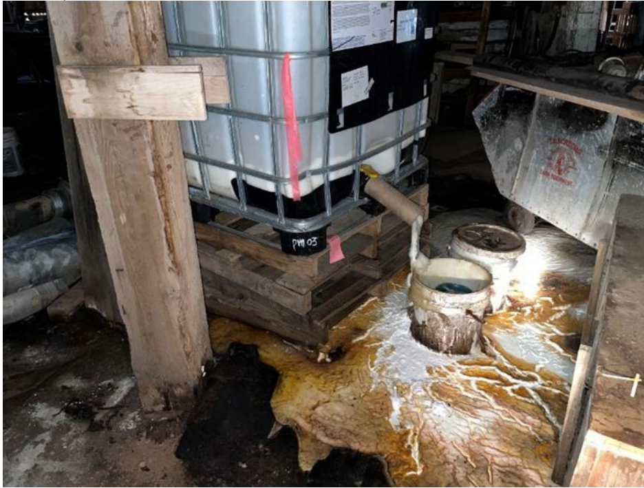
Figure 4: View of leaking tote.
