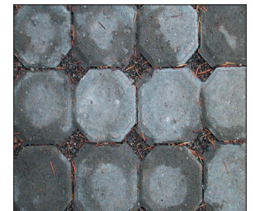
Top View of Porous Block Paving. Beveled corners allow for water to filter through to underlying soil
