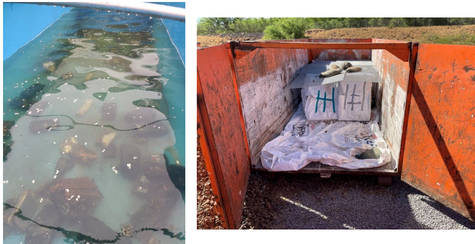
Figure 10. Pool with batteries? (LEFT photo) BESS/ESS power wall units collected from the Maui Wildfires are stored in tyvek wrapping to minimize spread of toxic ash . Expanded metal mesh is placed on top and weighted with sandbags to prevent energetic cylindrical cell launching, which could cause a brush fire (RIGHT photo).
