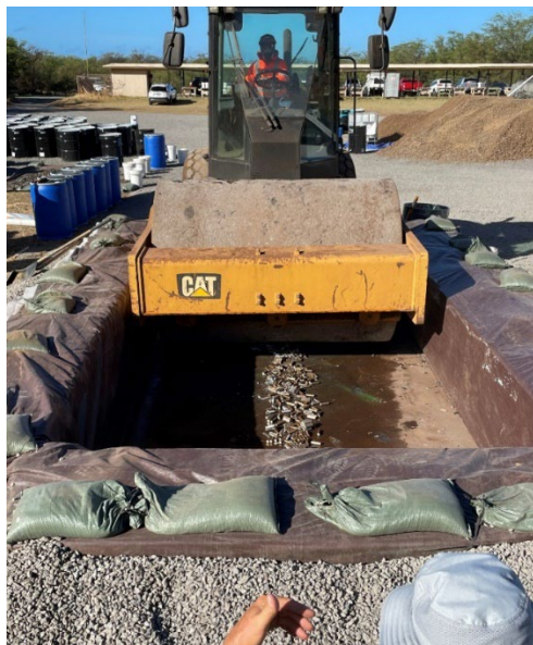
Figure 14. A still photo of deconstruction taking place.
