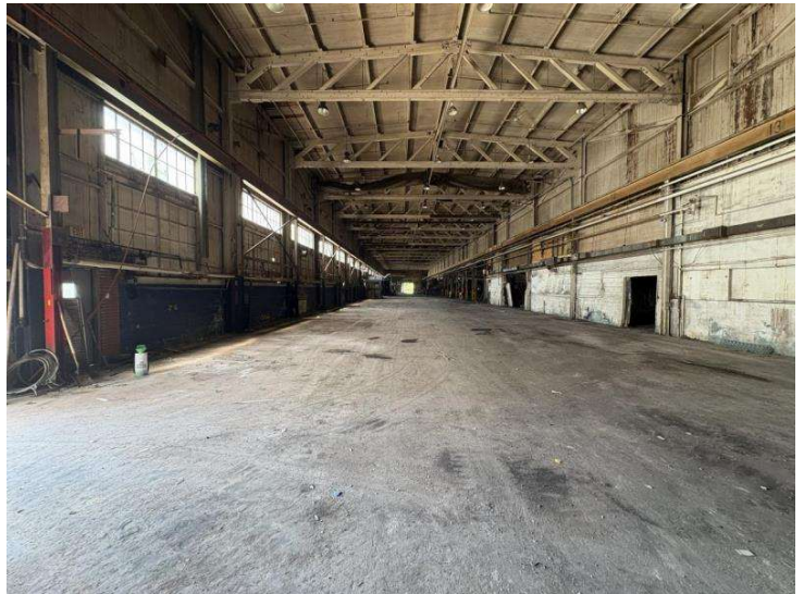
Post-removal image of the Omni Polymers Site
