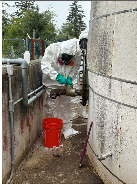
EPA contractor assessing the condition of a caustic tank valve.
