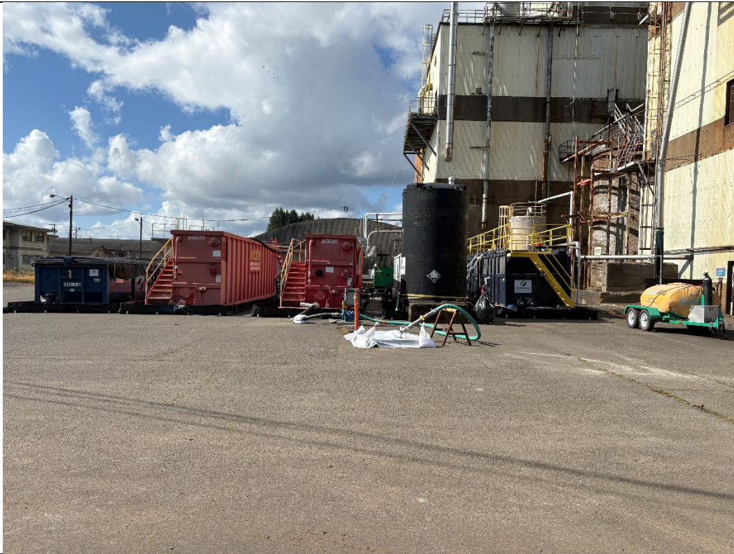
Fully constructed and operational waste treatment plant.
