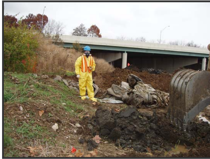
SITE: Alum Creek Bike Path Drum Site DATE: 11/8/2006 TIME: 1140 PHOTO NO: 7 DIRECTION: Northwest PHOTOGRAPHER: Anne Busher SUBJECT: START performing air monitoring during excavation activities.
