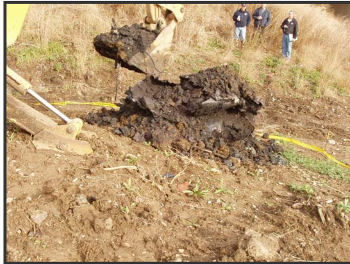
SITE: Alum Creek Bike Path Drum Site DATE: 11/8/2006 TIME: 0927 PHOTO NO: 1 DIRECTION: North PHOTOGRAPHER: Anne Busher SUBJECT: Fifty-five-gallon drum being unearthed from trench number 1.
