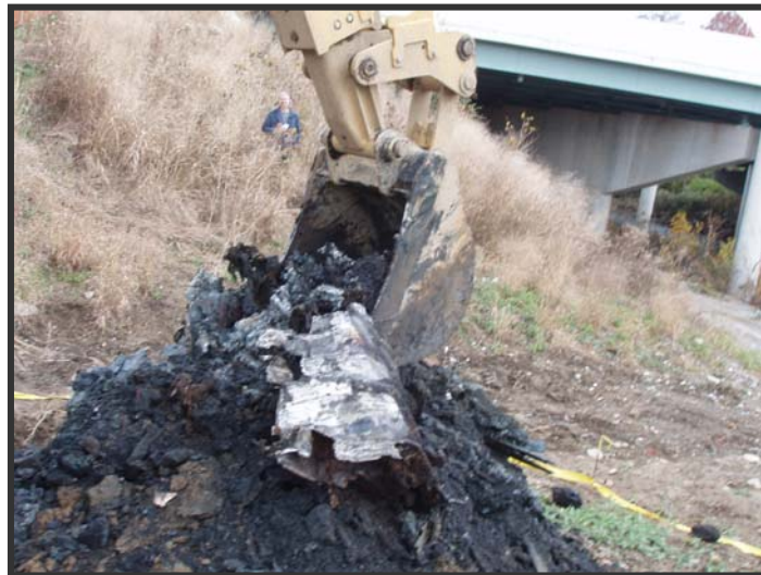
SITE: Alum Creek Bike Path Drum Site DATE: 11/8/2006 TIME: 0935 PHOTO NO: 2 DIRECTION: NE PHOTOGRAPHER: Anne Busher SUBJECT: A second 55-gallon drum being unearthed from trench number 1.
