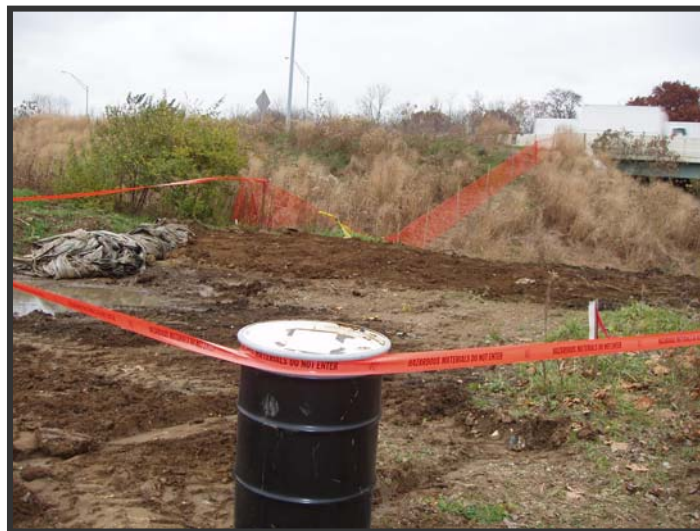
SITE: Alum Creek Bike Path Drum Site DATE: 11/8/2006 TIME: 1405 PHOTO NO: 8 DIRECTION: North PHOTOGRAPHER: Anne Busher SUBJECT: The site following excavation activities.
