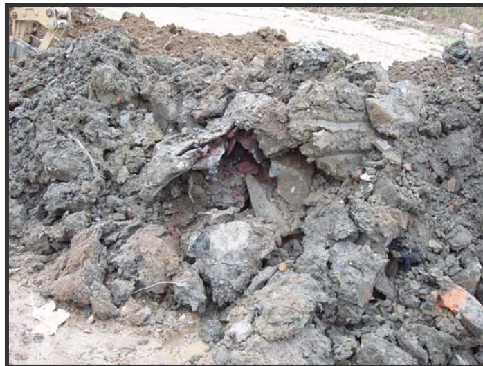
SITE: Alum Creek Bike Path Drum Site DATE: 11/8/2006 TIME: 1156 PHOTO NO: 4 DIRECTION: North PHOTOGRAPHER: Anne Busher SUBJECT: A 55-gallon drum unearthed from trench number 3.
