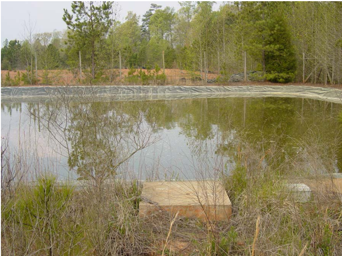
Figure 54. Photograph of the Process Plant Carbon Pond. The electric pump has been removed from its concrete base.
