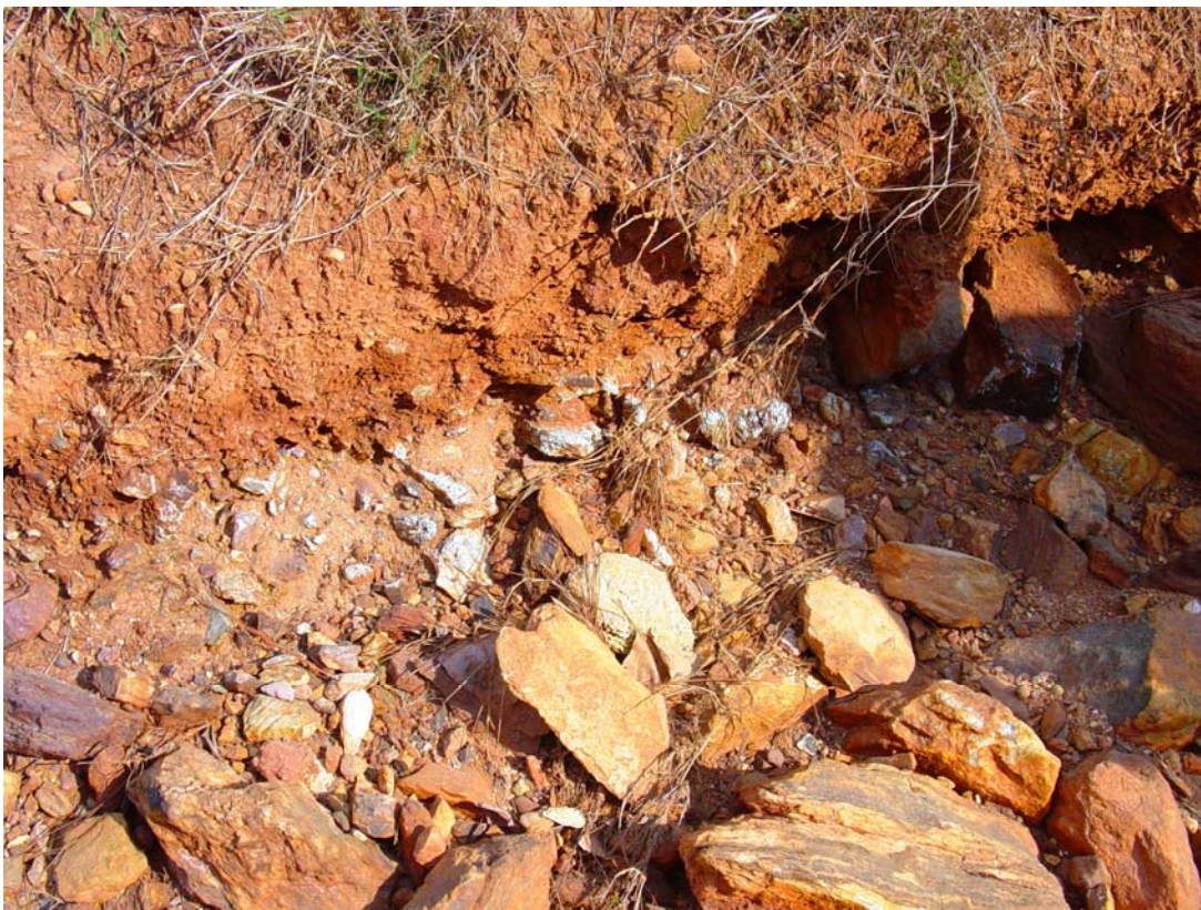
Figure 57. Damp soil at the seepage line along the toe of the fill embankment supporting the Process Plant Contingency Pond. Note the prussian blue coating the rocks below the damp soil.
