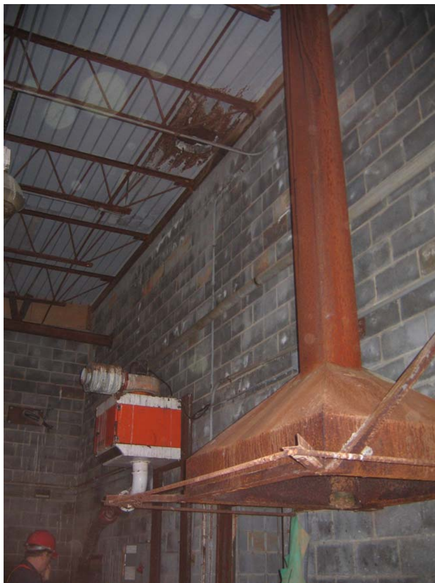
Figure 40. Two fume ventilation systems used for the fire assay process. At left is a portion of the fume ventilation system for the small melting/assay furnace, at right is the fire assay acid fume hood and ventilation duct leading to the roof.
