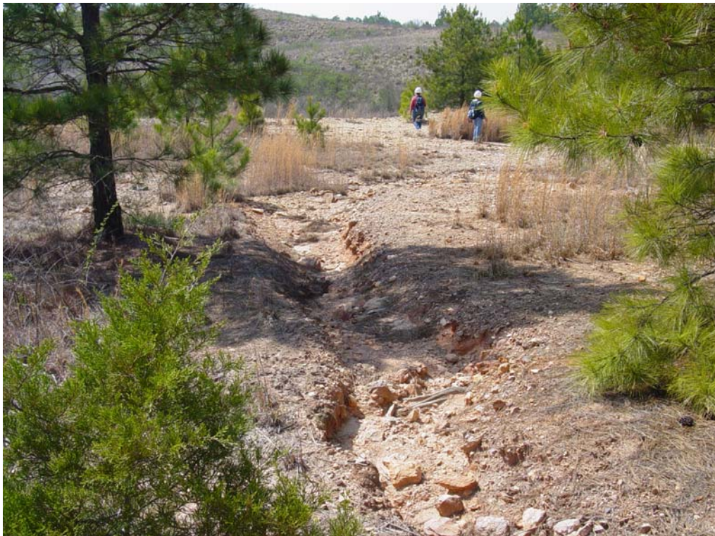
Figure 25. Shallow erosion gully formed in an un-reclaimed area on the gently sloping top of the Industrial Solid Waste Landfill.
