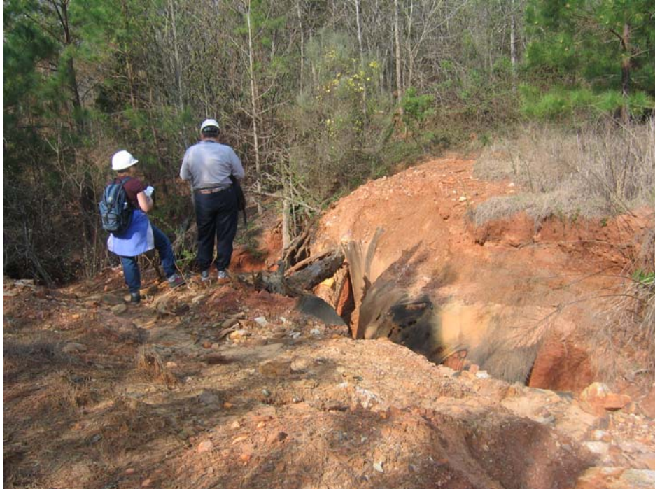
Figure 64. Failed sediment control structure on eroded diversion ditch near the Process Plant Contingency Pond.
