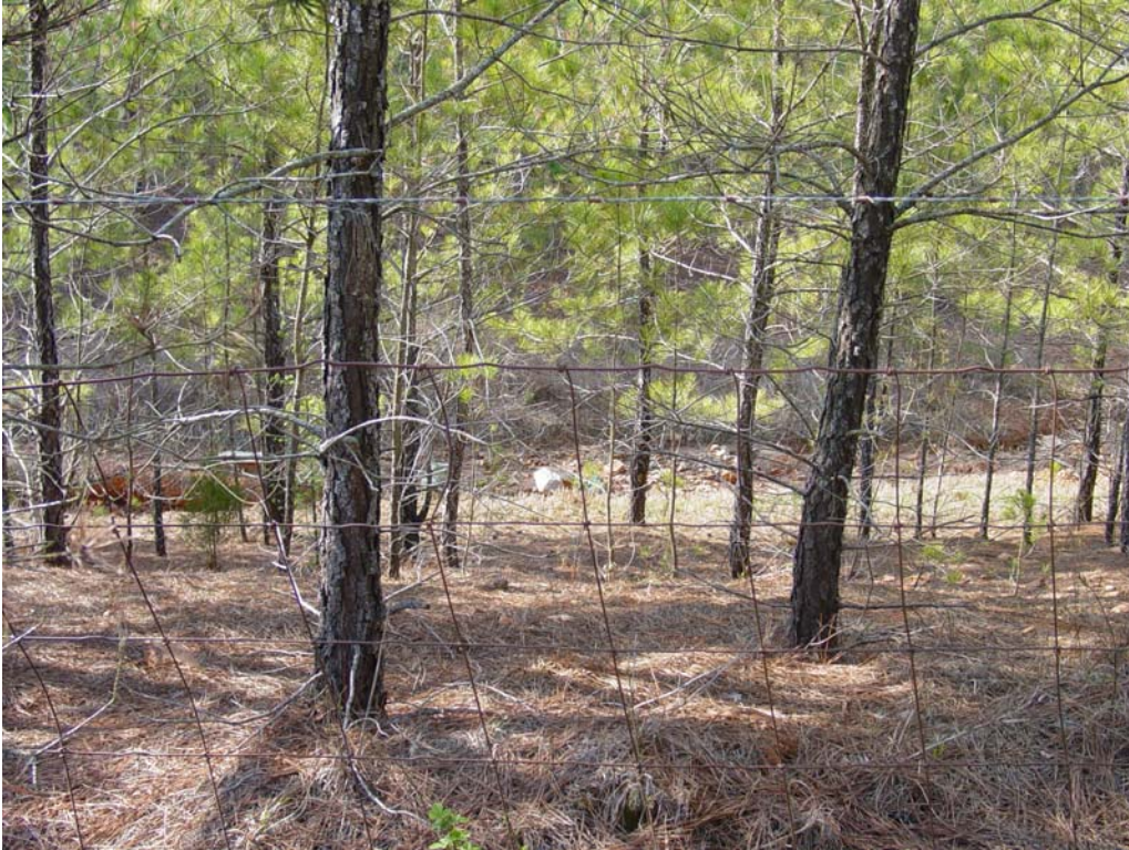
Figure 5. Close up view of fencing around the Process Plant Contingency Pond showing a smooth-wire grid and an upper single strand of barbed wire.
