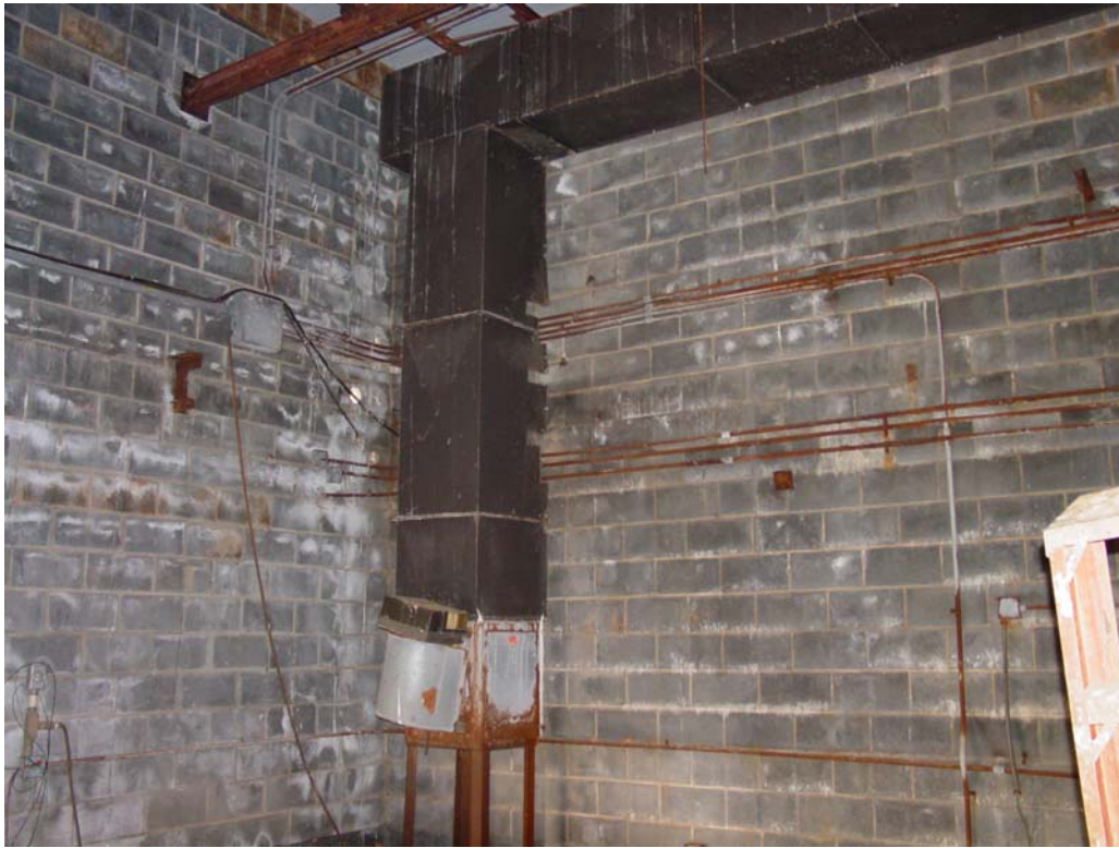
Figure 41. Ducting for large fume ventilation system used during gold production.
