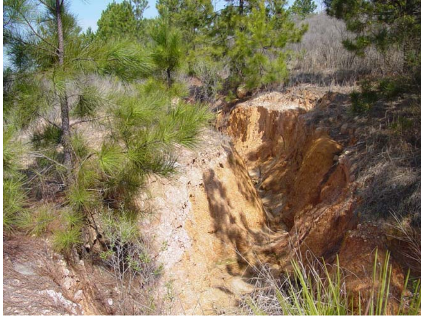
Figure 65. Erosion of diversion ditch adjacent to the Industrial Solid Waste Landfill.
