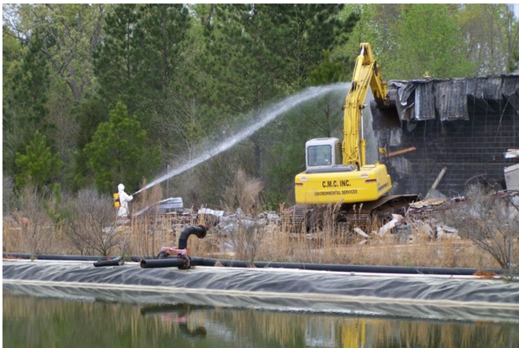
Figure 42. Demolition of the Gold Assay and Melting Furnace Building on March 30, 2007 as part of the Emergency Response.
