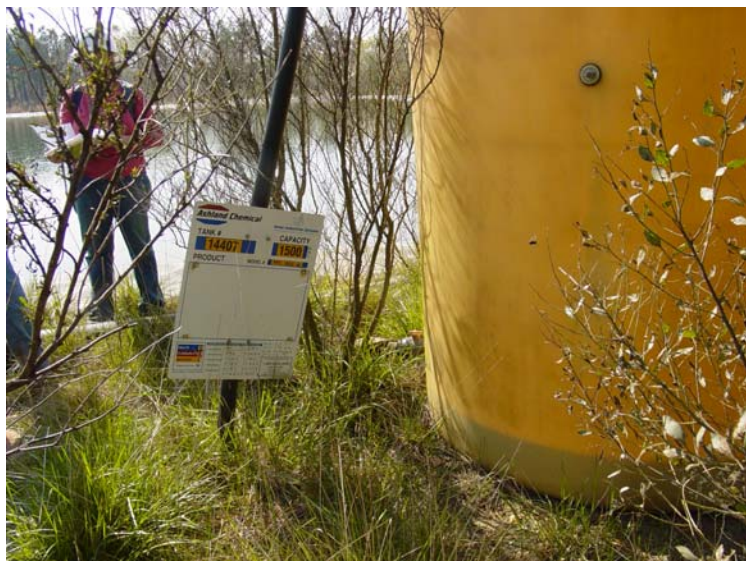
Figure 47. Tank next to the Permanent Heap Barren Pond was used for make up cyanide solution. The fluid was sampled for analysis by others.
