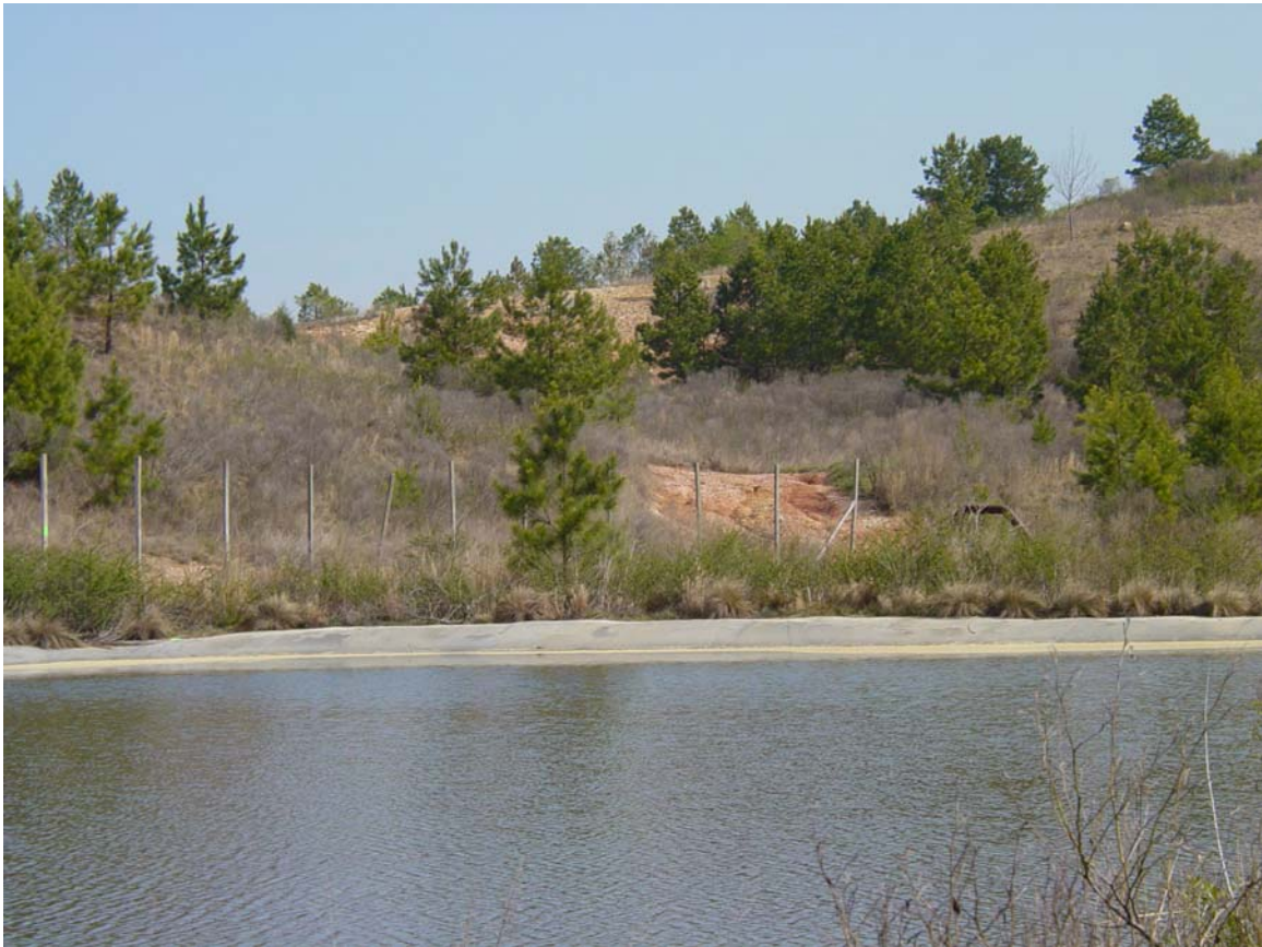
Figure 59. View of the Permanent Heap Rinse Pond. The disturbed area just above the pond is the location of a major acid seep from the Permanent Heap Leach Pad which is lowering the pH of this pond.
