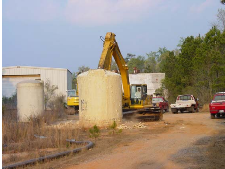
Figure 46. Removing foam insulation from the 3,000 gallon tank containing caustic prior to taking it to the pit. Another tank is seen to the left.
