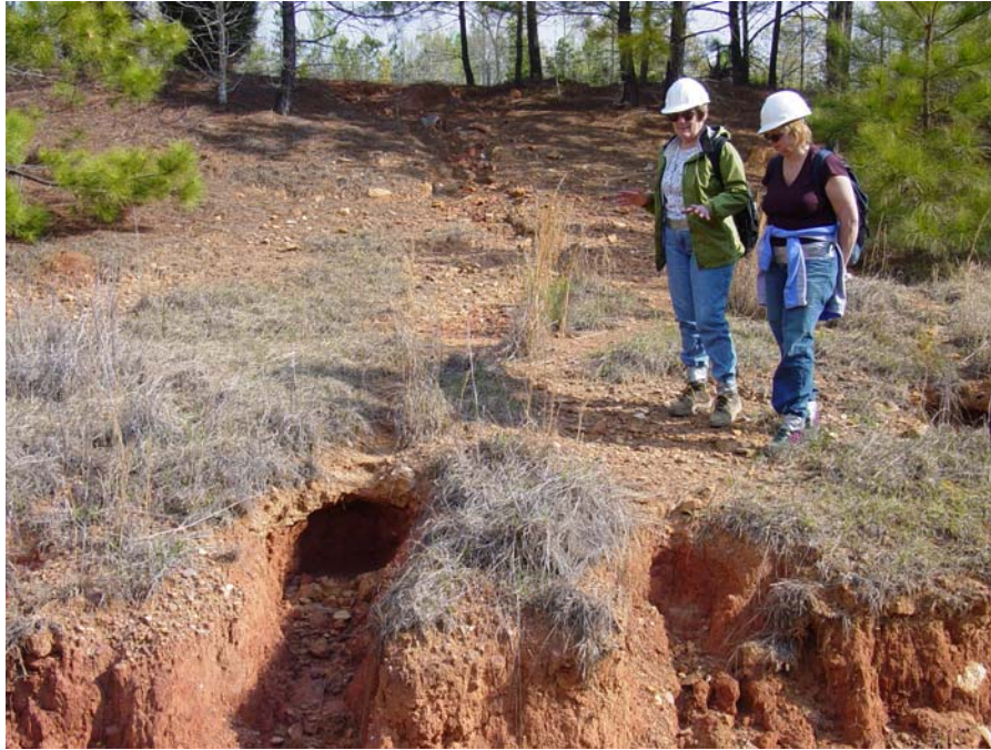
Figure 56. Signs of erosion and piping of the outslope of the fill embankment supporting the contingency pond.
