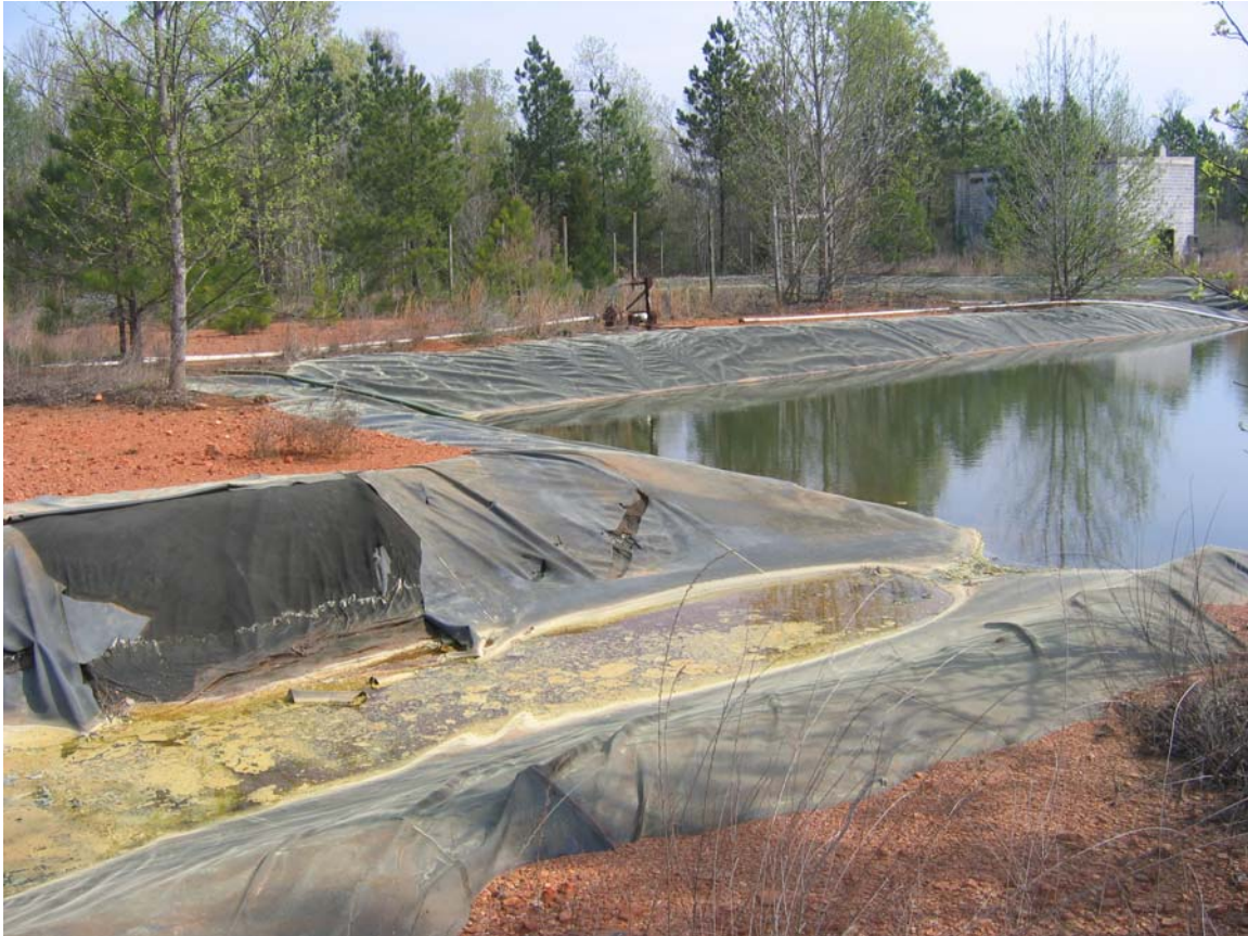
Figure 53. Discharge channel and the west portion of the Process Plant Rinse Pond. This pond, like those upstream of it, is full, all additional precipitation results in discharge to the unlined Process Plant Contingency Pond.
