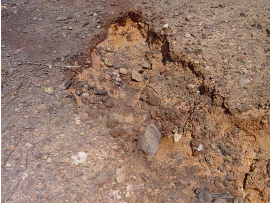
Figure 26. Seepage discharging from near the bottom of the slope of the west side of the Industrial Solid Waste Landfill.
