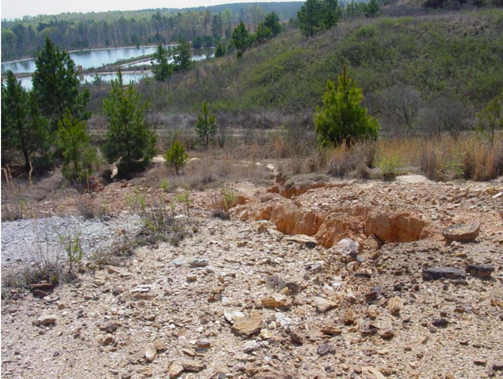
Figure 24. Deeply incised erosion gully in un-reclaimed slope of the Industrial Solid Waste Landfill.
