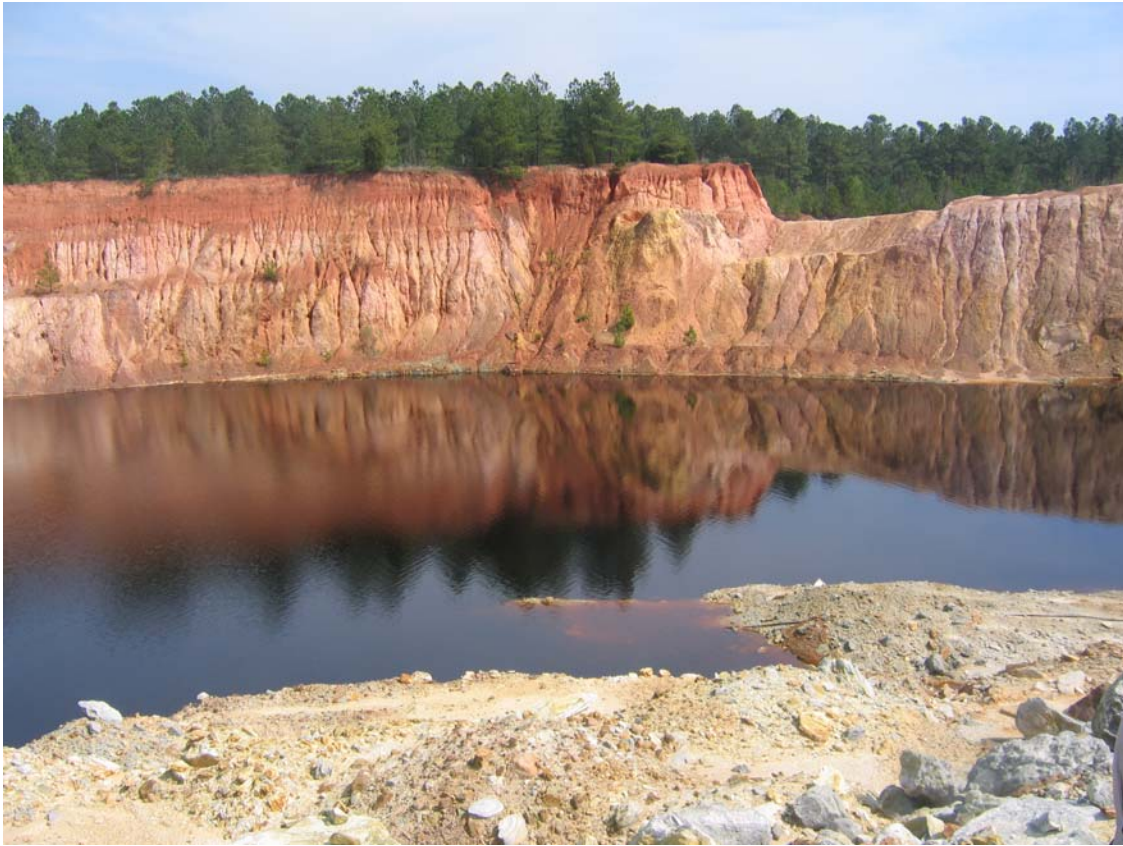
Figure 10. Photograph looking towards east side of the pit. The east highwall area shows signs of volunteer vegetation and it likely has a relatively low permeability. In the upper right part of the photograph, the excavation from the clay borrow area can be seen which removed the top layer of red-colored clay soil.
