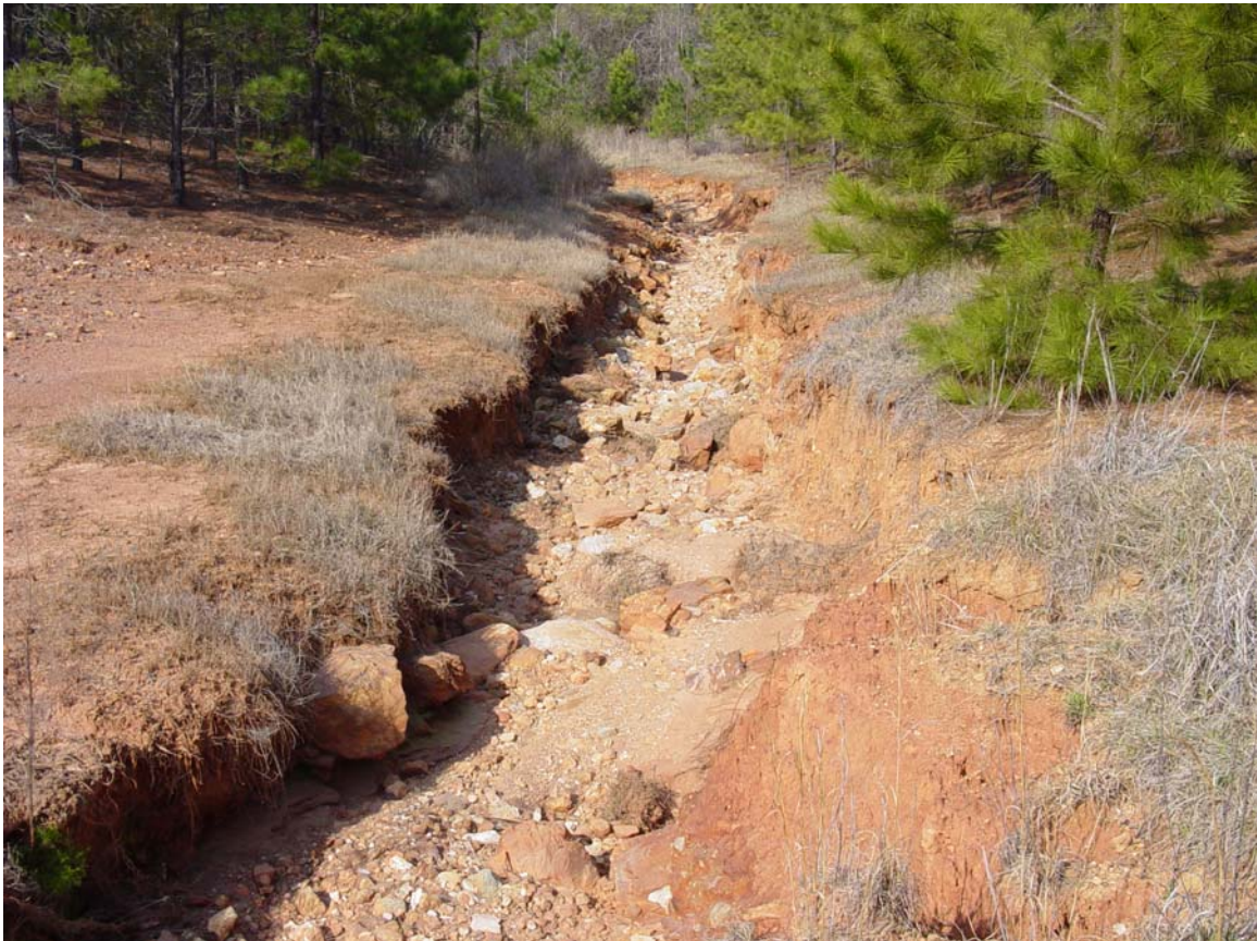
Figure 21. View to the west of the eroded diversion ditch on the north side of Waste Rock Disposal Area A. Significant amounts of pyrite rich waste rock are present in this eroded channel which is likely a source of acid drainage.
