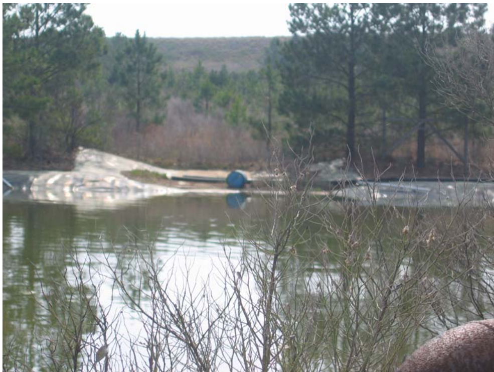
Figure 34. Photograph looking across the Plant Pregnant Pond showing the geomembrane-covered seepage outlet from the Reusable Heap Leach Pad.
