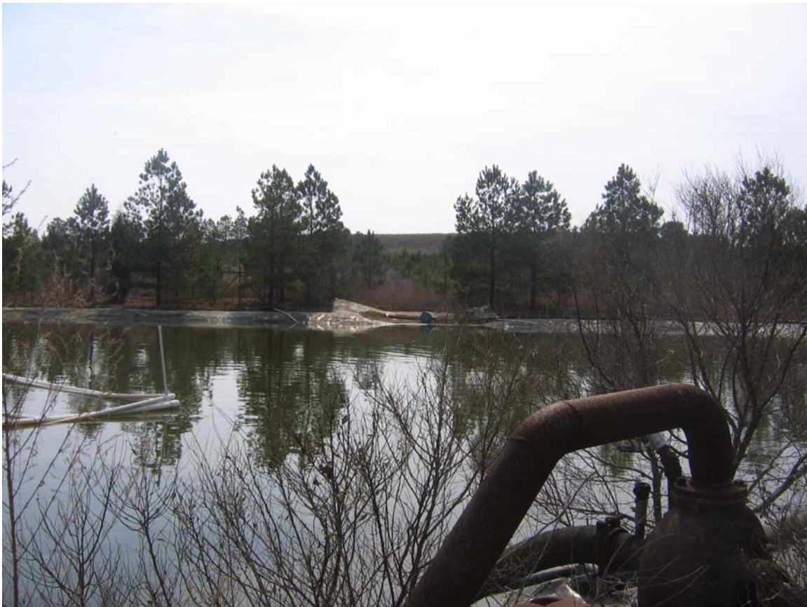
Figure 51. Photograph of the Process Plant Pregnant Pond. The view across the pond shows the seepage inflow area from the Reusable Heap-Leach Pad. An electric pump can be seen at lower right.
