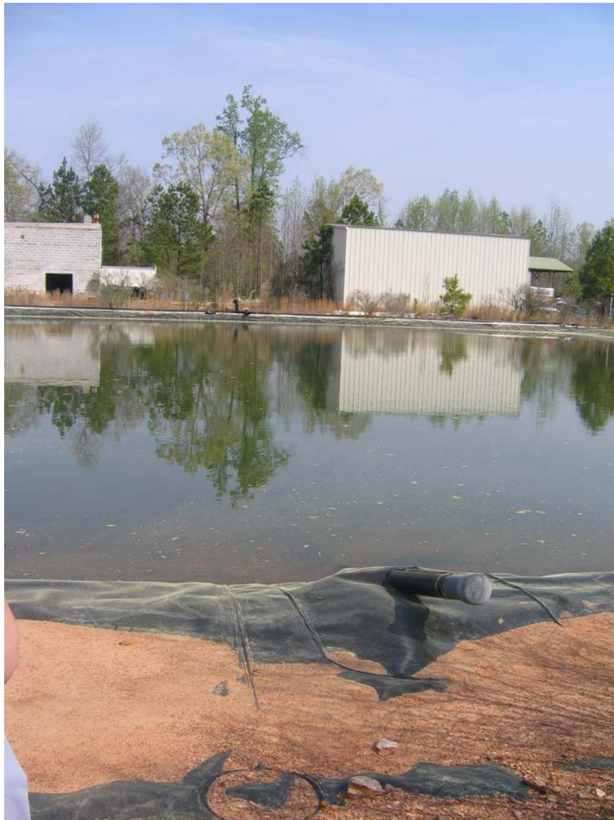
Figure 52. Photograph showing the Process Plant Barren Pond and leak detection sump riser pipe.
