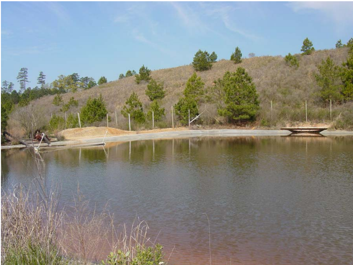
Figure 58. Photograph of the Permanent Heap Pregnant Pond looking towards the west. The southwest portion of the capped and reclaimed Permanent Heap forms the hillside in the background of the photograph. Note the small pile of acidic material adjacent to the pump station on the left side of the photograph.
