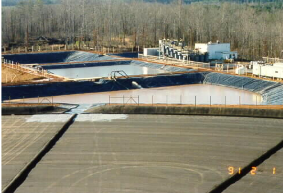
Figure 33. Photograph showing the Reusable Leach Pad (lower half of photograph) at the Barite Hill mine prior to ore placement in 1991 (From the Scotia International Website). Note how the pad is designed to discharge cyanide solution seepage to the Plant Pregnant Pond.
