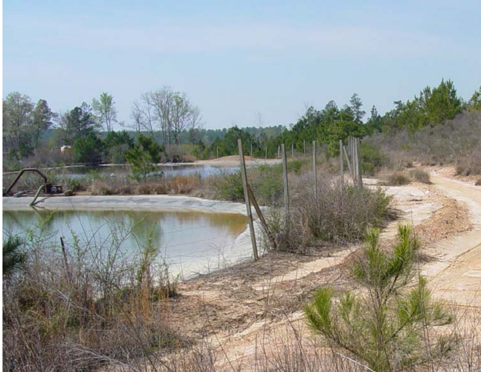
Figure 6. Photograph showing a transition in the fencing at the Permanent Heap Rinse Pond. At left is a three strand barbed wire fence, at right is the taller fence with a smooth wire grid and upper strands of barbed wire.
