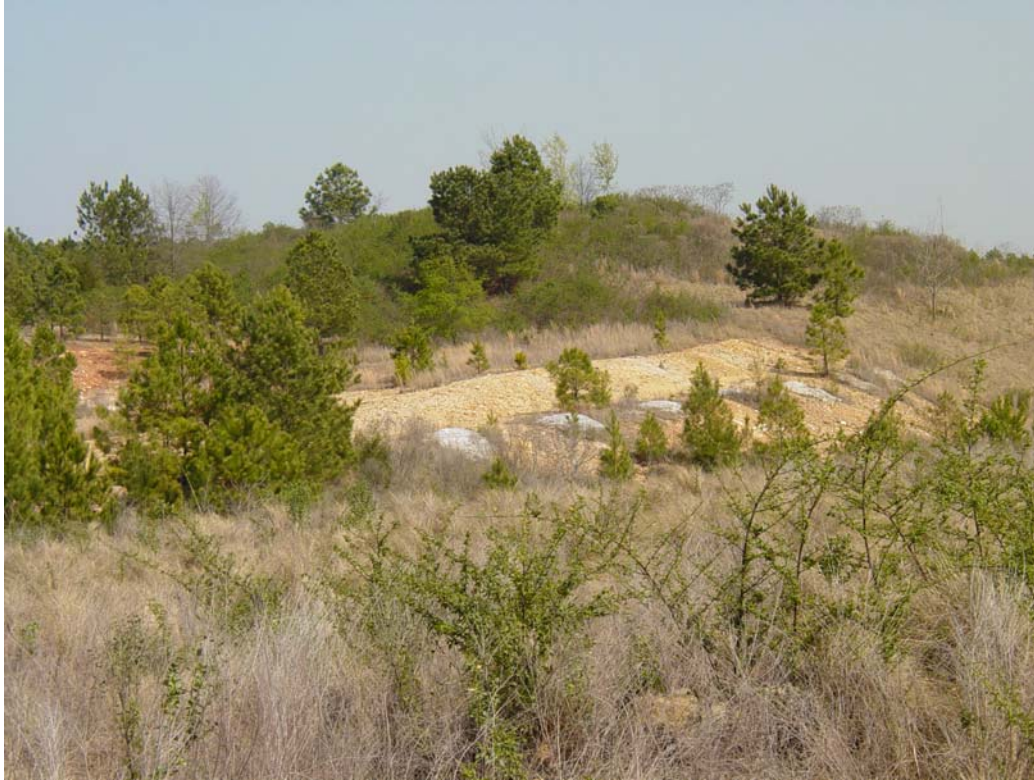
Figure 23. View of incomplete reclamation on the west side of the Industrial Solid Waste Landfill. Note that organic matter (brown ring around white piles) and slaked lime (white piles) have been dumped but were not spread and incorporated into the mine waste. One deep erosion gully (see Fig. 24) cuts down through this unreclaimed slope to the right and a shallow gully (see Fig. 24) is eroding the unreclaimed area on the left side of the photograph.
