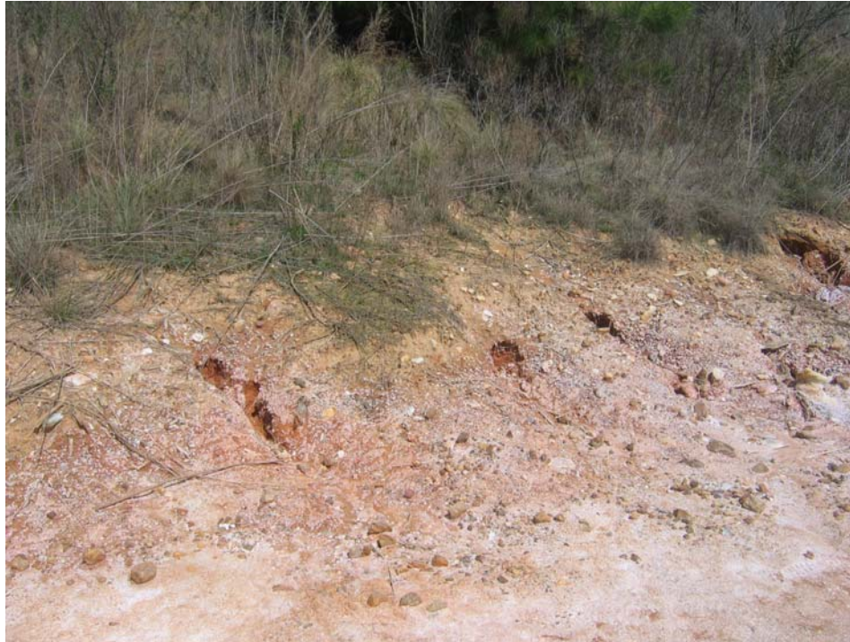
Figure 28. Acid seepage killing vegetation and causing piping like internal erosion at the south toe of the Permanent Heap Leach Pad.
