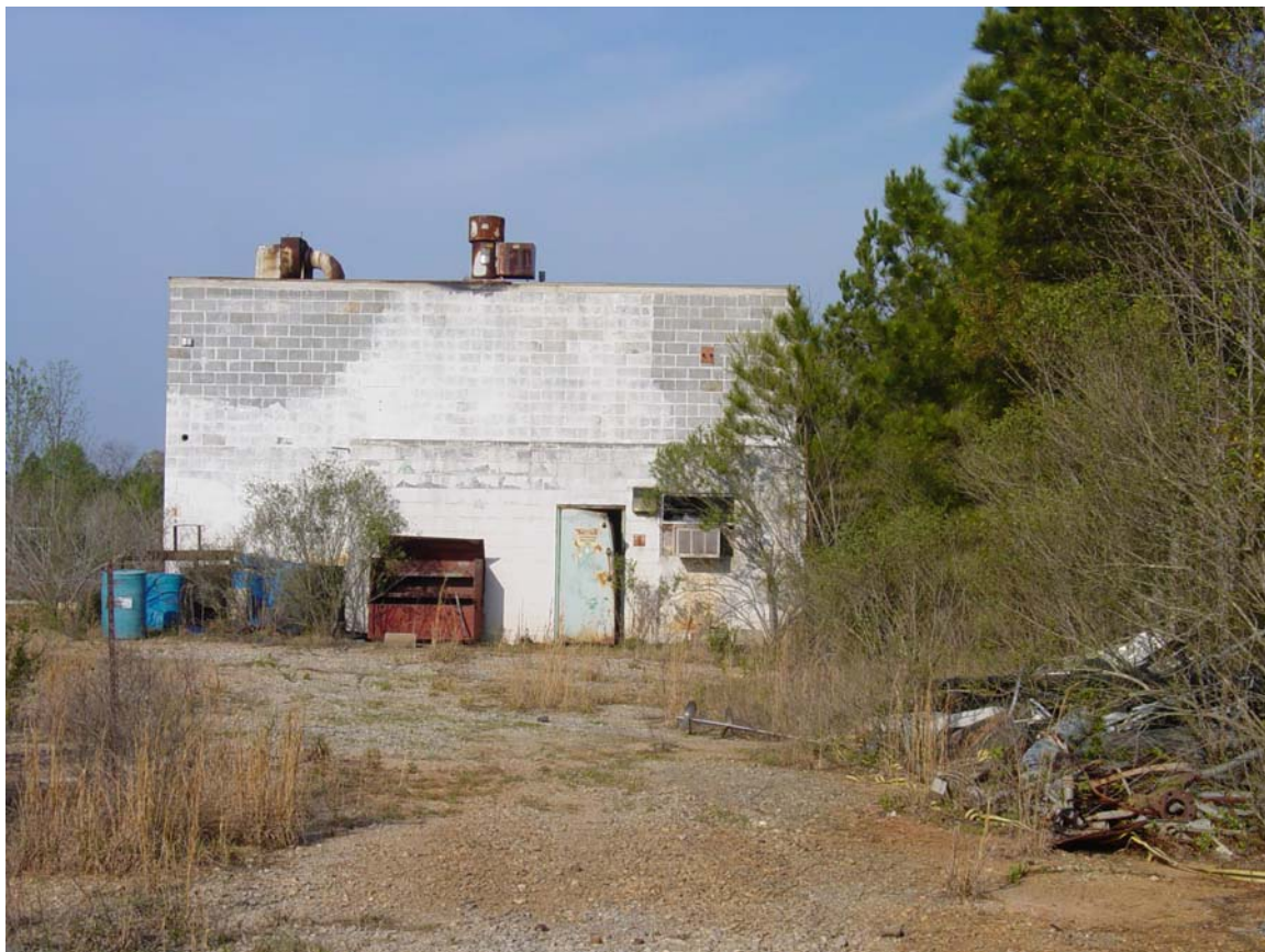
Figure 39. The gold assay and melting furnace building. Note fume ventilation system components on the roof.
