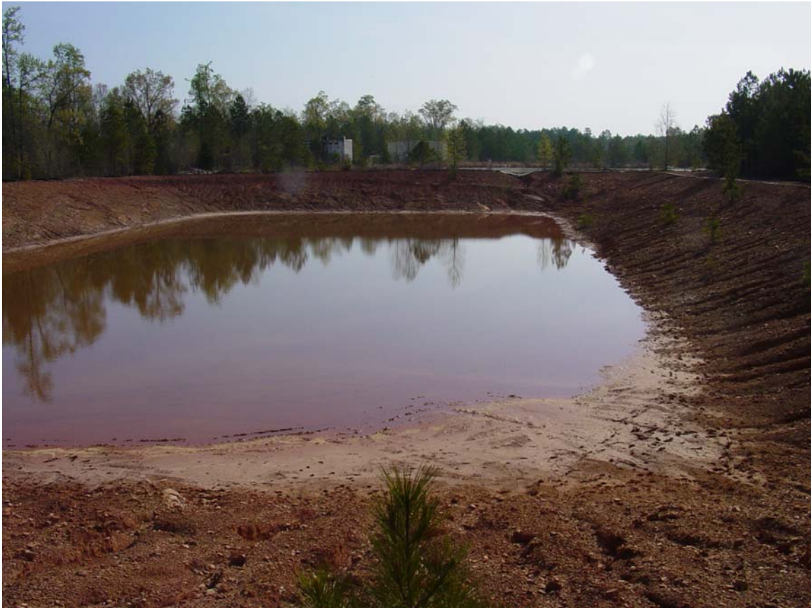
Figure 55. View of the Plant Contingency Pond (view looking towards the west). Note that the liner has been cut and removed. The slope in the right side of the photograph is weathered bedrock. The slope in the left side of the photograph is a fill embankment through which water is seeping.
