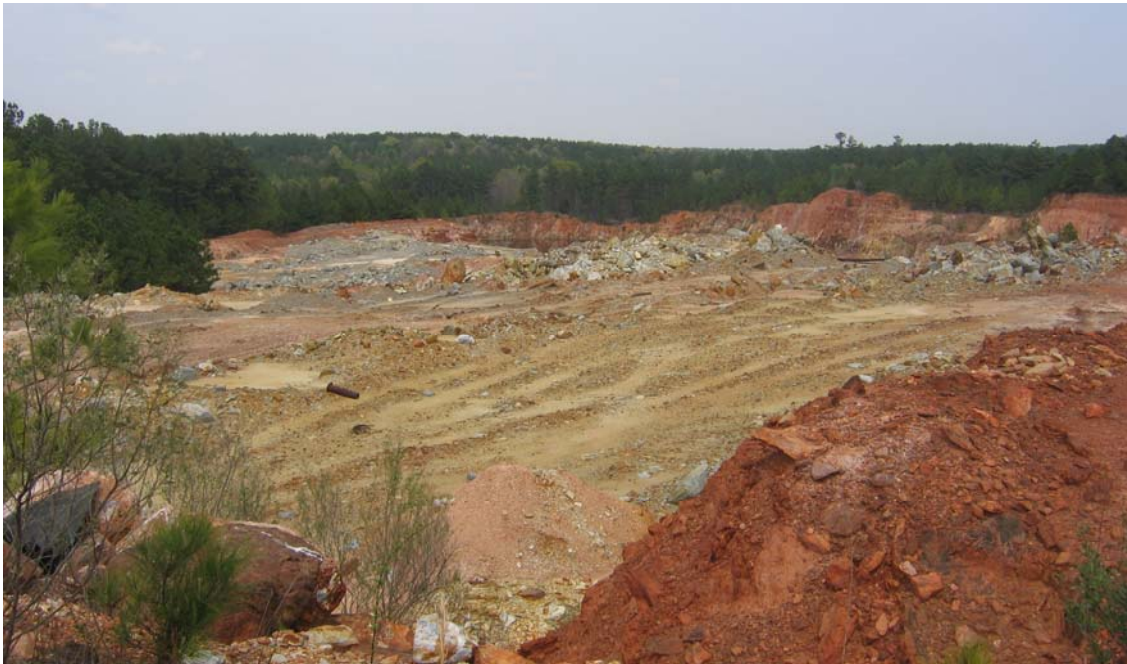
Figure 14. Photograph showing the disturbed area on the southwest side of the Barite Hill Pit. This is a major source area for acid water draining into the pit.
