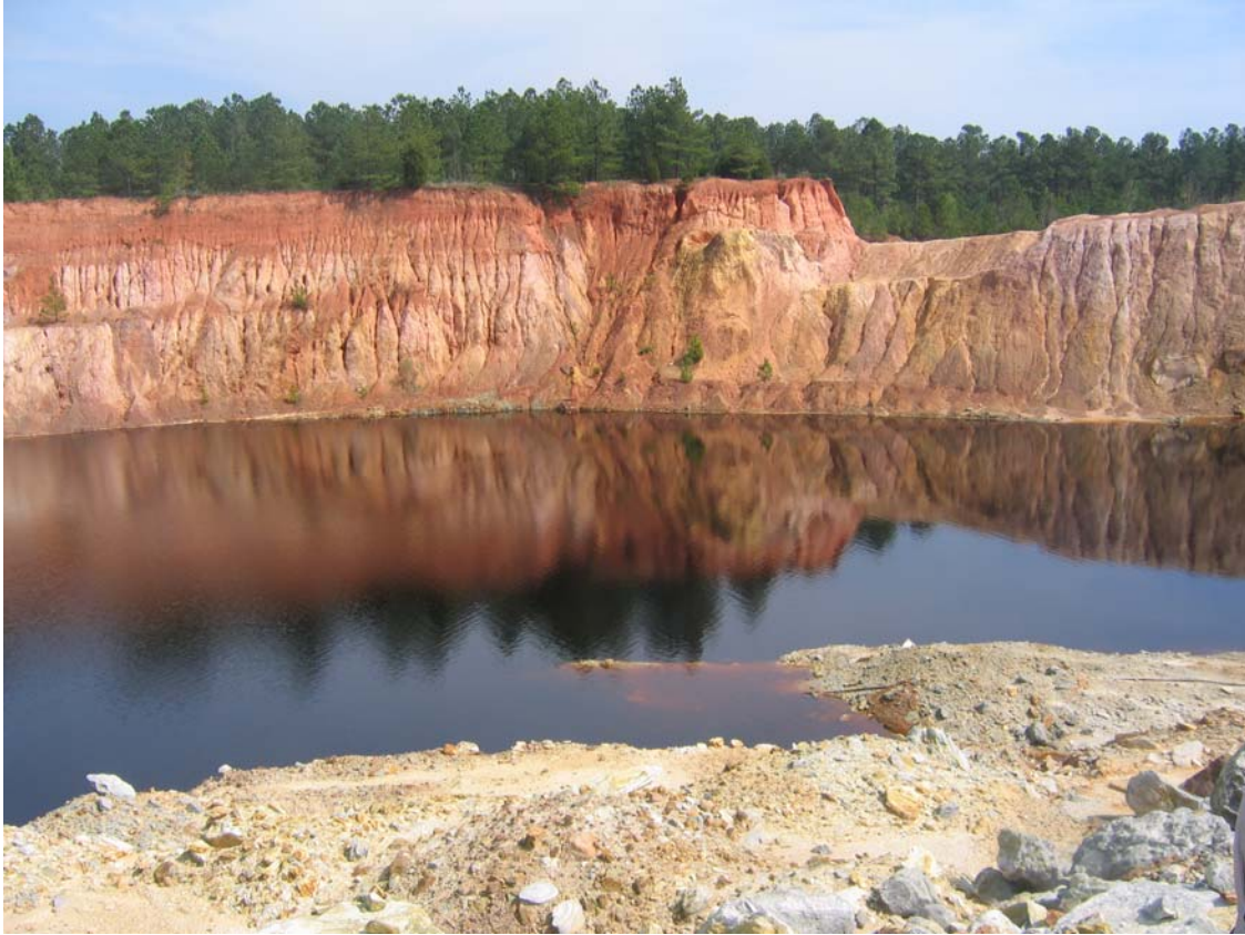
Figure 3. Photograph looking towards east side of the pit. The east highwall area shows signs of volunteer vegetation and it likely has a relatively low permeability. In the upper right part of the photograph, the excavation from the clay borrow area can be seen which removed the top layer of red-colored clay soil.
