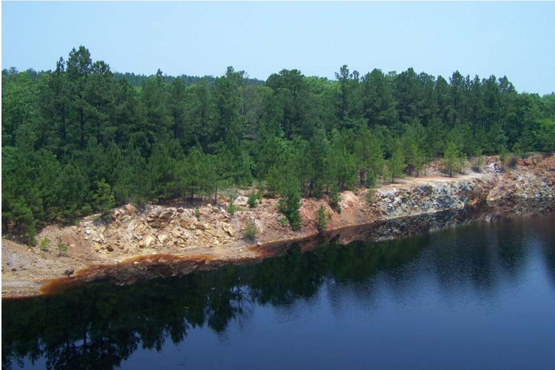
Figure 9. View of the north pit wall where outflow from the pit will eventually occur. The spill point is likely to be near the left side of the photograph.
