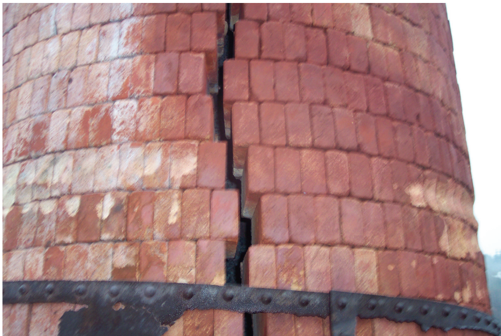
Photo #7 View of 1-1/2" to 2" opening size of south side crack.
