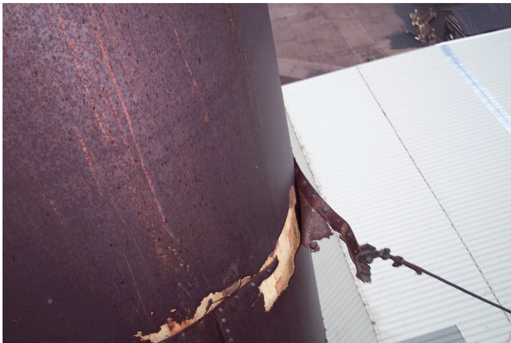
Photo #11 View of “failed” northwest guy wire cable connection.
