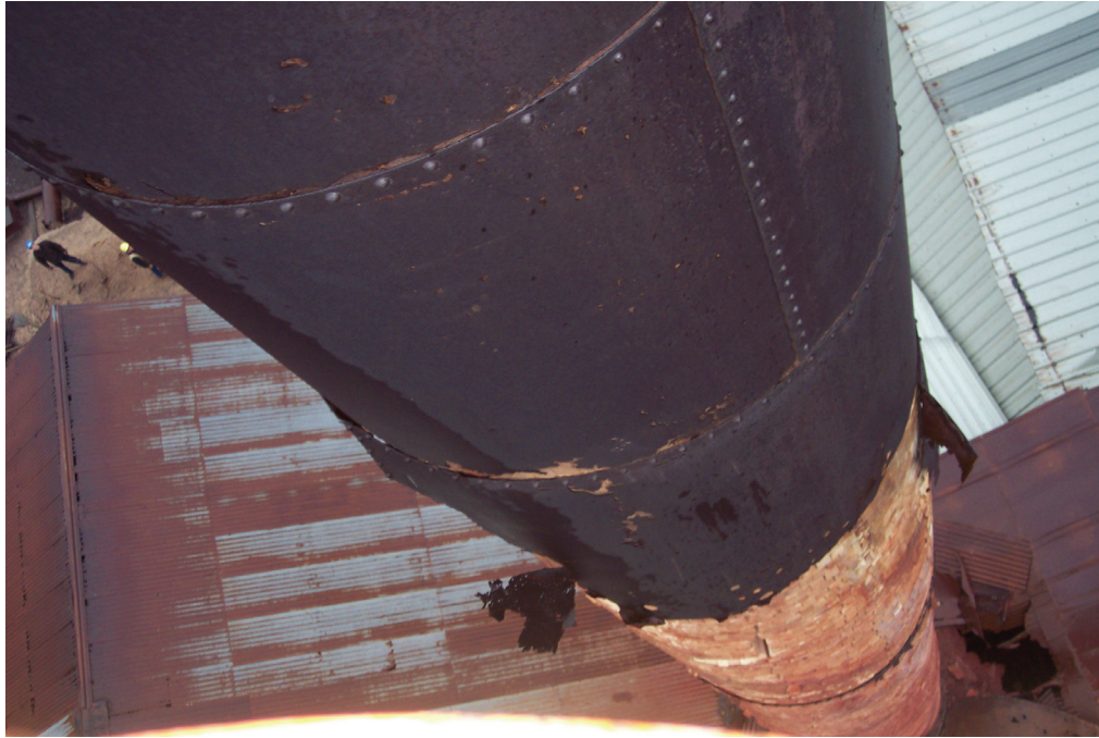
Photo #13 View of remaining steel shell of stack on north side.
