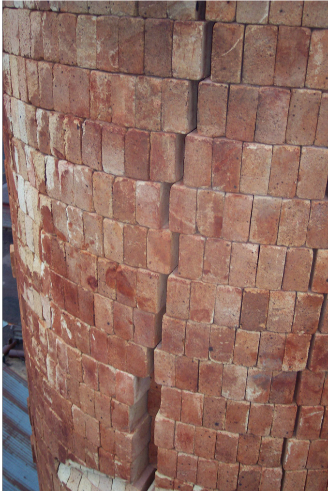
Photo #14 View of cracks in stack forming on the north side.
