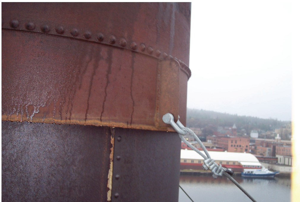
Photo #12 View of new guy wire cable on temporary stack cap just above.
