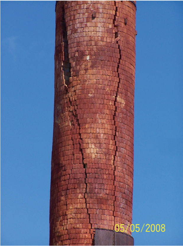
Photo #4 View of converging south and southwest cracks.
