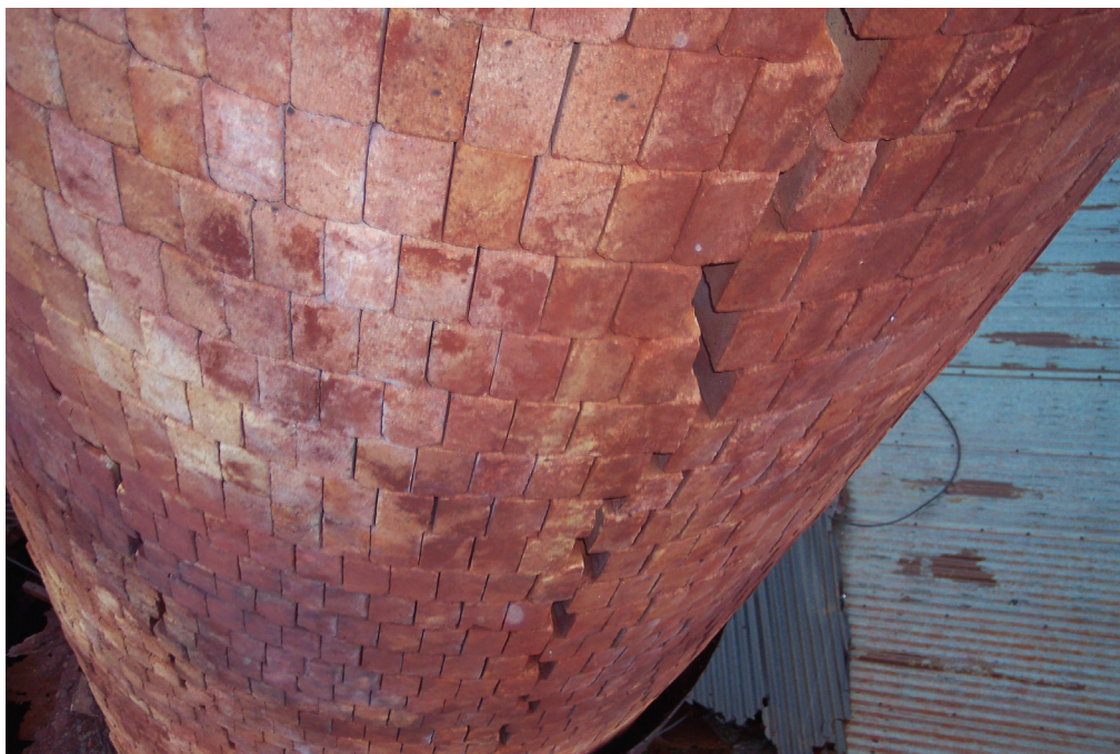
Photo #8 View looking down at both the south and southwest side crack. Circular stack shape starting to become "egg-shaped".
