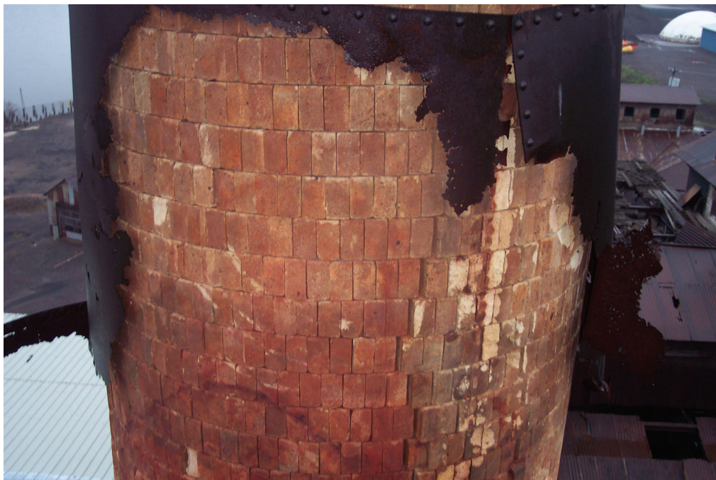
Photo #9 View of deteriorating steel shell and crack on east side.
