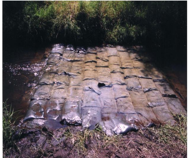
The portable dam pictured above was installed along the Blackstone Canal in preparation of EPA removal actions.
