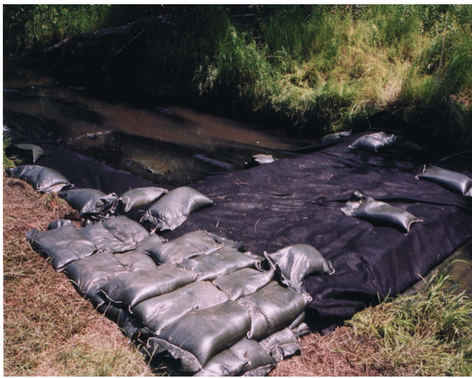
The portable dam pictured above was installed along the Blackstone Canal in preparation of EPA removal actions.
