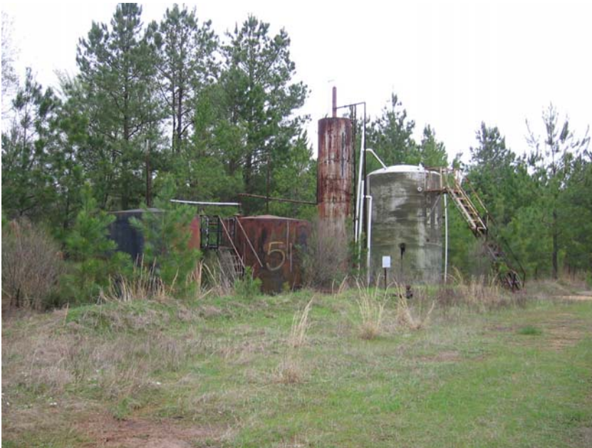
Site Name: Quality Petroleum, Inc.-Hoffman, et al. Project No.: E06614 Photo No.: 0101 Direction: NW Contract No. Date: 04/01/2008 Time: 1:20:00 PM Photographer/Witness: Farrar, Will/N/A Description: E06614: AST1 through AST3 and S1 in CONT1.
