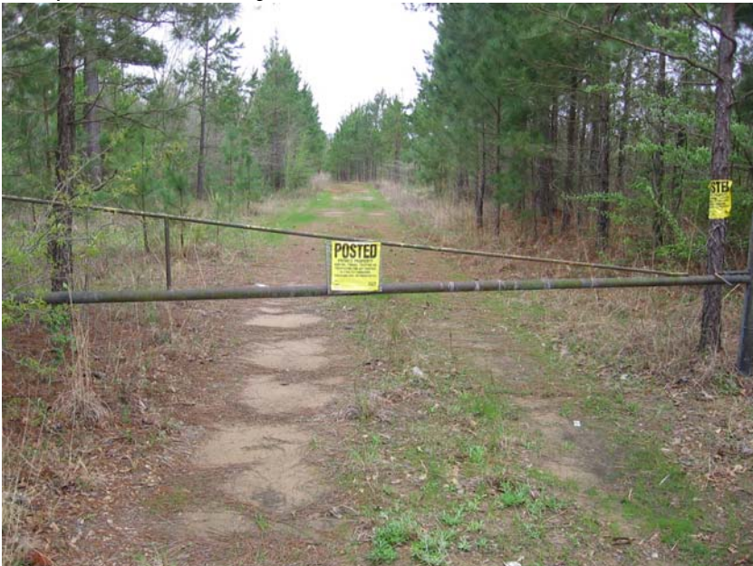
Site Name: Quality Petroleum, Inc.-Hoffman, et al. Project No.: E06614 Photo No.: 0103 Direction: SSE Contract No. Date: 04/01/2008 Time: 1:21:00 PM Photographer/Witness: Farrar, Will/N/A Description: E06614: Unlocked gate across access road to facility.
