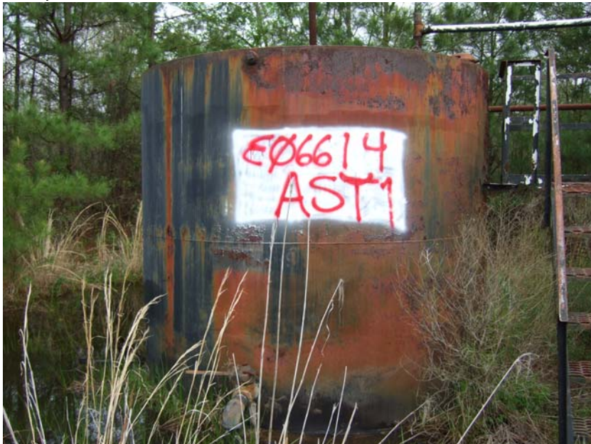
Site Name: Quality Petroleum, Inc.-Hoffman, et al. Project No.: E06614 Photo No.: 0203 Direction: W Contract No.: Date: 04/05/2008 Time: 9:33:00 AM Photographer/Witness: Sekerka, Robert/Johnson, Colin Description: E06614: Label on AST1.
