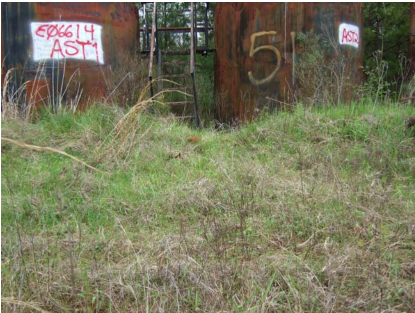
Site Name: Quality Petroleum, Inc.-Hoffman, et al. Project No.: E06614 Photo No.: 0223 Direction: W Contract No. Date: 04/05/2008 Time: 10:15:00 A Photographer/Witness: Sekerka, Robert/Johnson, Colin Description: E06614: Shallow breach on southeast berm of CONT1.
