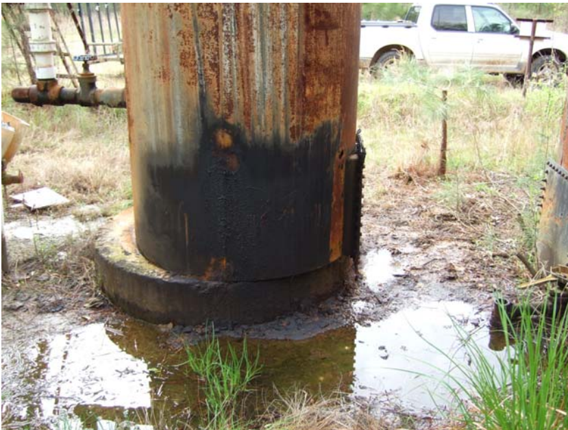
Site Name: Quality Petroleum, Inc.-Hoffman, et al. Project No.: E06614 Photo No.: 0213 Direction: E Contract No.: Date: 04/05/2008 Time: 9:41:00 AM Photographer/Witness: Sekerka, Robert/Johnson, Colin Description: E06614: Rust, corrosion and delaminated metal at base of S1 and evidence of prior oil release.
