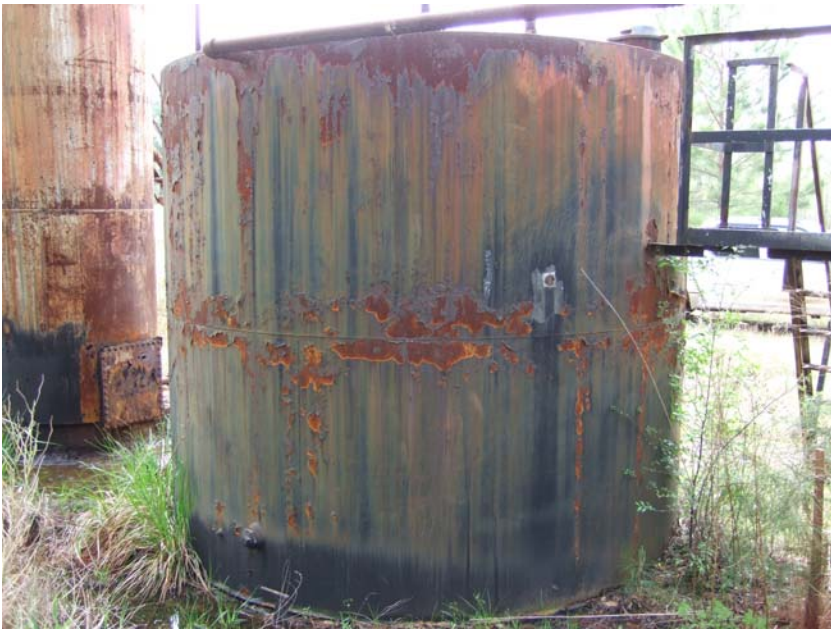
Site Name: Quality Petroleum, Inc.-Hoffman, et al. Project No.: E06614 Photo No.: 0210 Direction: E Contract No.: Date: 04/05/2008 Time: 9:39:00 AM Photographer/Witness: Sekerka, Robert/Johnson, Colin Description: E06614: Rust, corrosion and delaminated metal on AST2.
