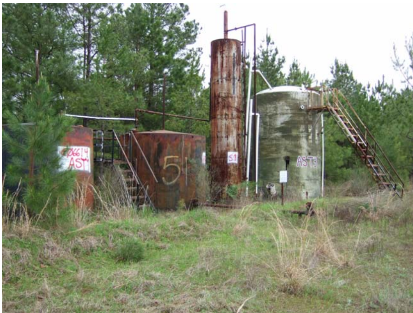
Site Name: Quality Petroleum, Inc.-Hoffman, et al. Project No.: E06614 Photo No.: 0201 Direction: NW Contract No.: Date: 04/05/2008 Time: 9:28:00 AM Photographer/Witness: Sekerka, Robert/Johnson, Colin Description: E06614: AST1, AST2, AST3, and S1 in CONT1.
